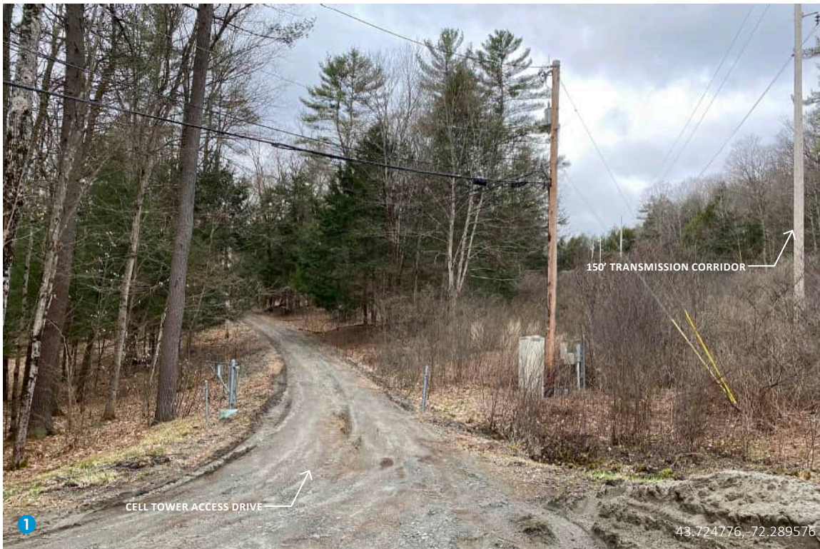
Photo 1: View from the entrance to the existing access road on Upper Loveland Road looking southwest toward the Project.
