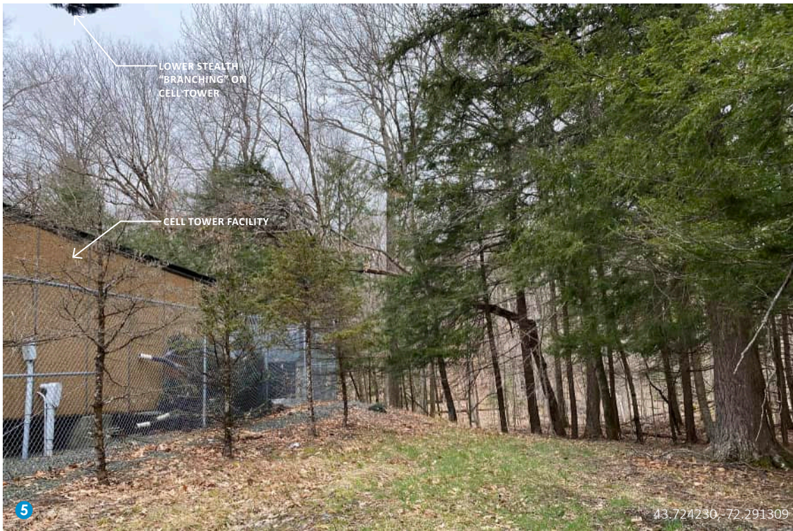
Photo 5: View from the end of the existing cell tower access road looking northwesterly toward the northern end of the Project. The cell tower facility is visible on the left side of the photo.
