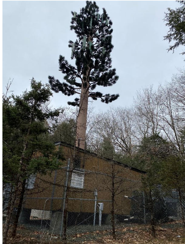
Image 8. View of the cellular communications tower facility adjacent to the Project.
