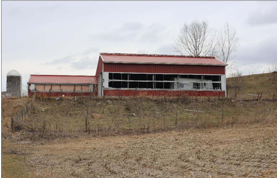
Looking north from the western edge of the solar site toward one of the adjacent farm buildings. The fence line of the solar array will basically follow the old farm fence visible in the foreground here. The main dairy complex is just beyond to the northwest (notice the silo on the left).
