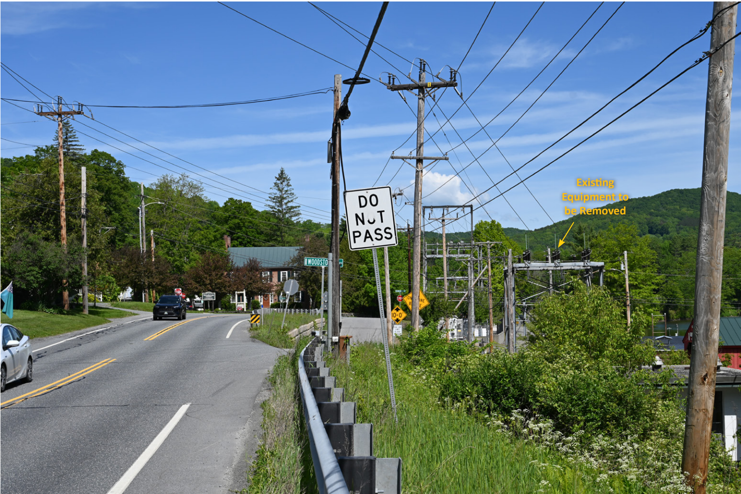
Viewpoint 6: View from Route 4, looking northwest towards existing infrastructure to be removed and proposed GSU transformer location. (50mm)
