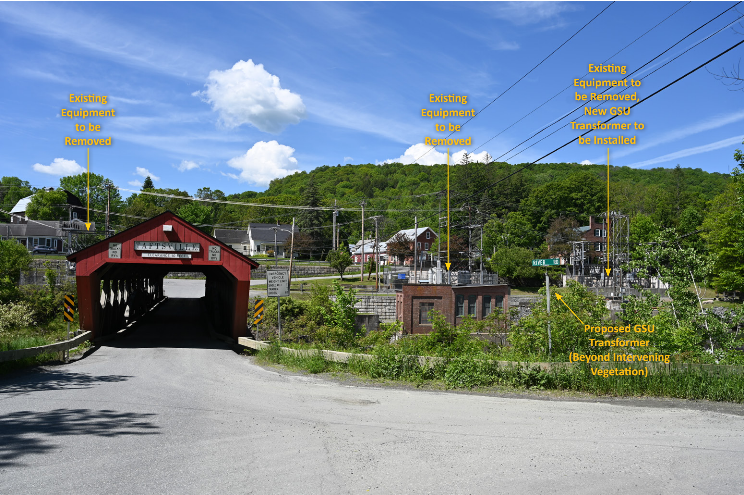
Viewpoint 11: Wide-angle view from the northeast side of the Taftsville Bridge looking southwest towards the existing substation infrastructure. (32.5mm)
