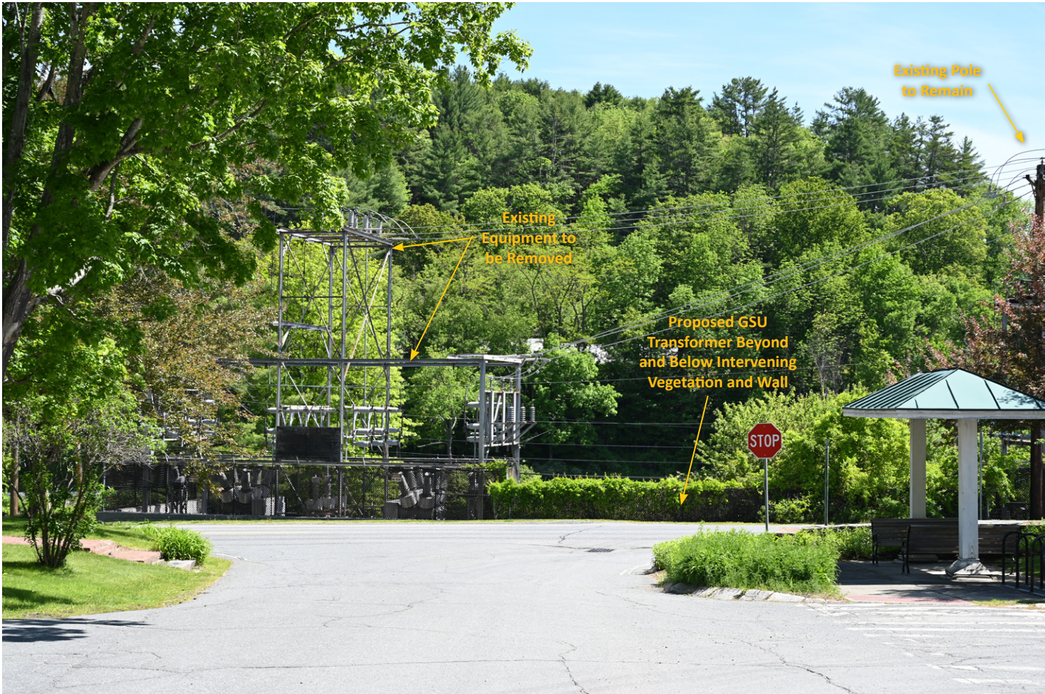
Viewpoint 9: View from Happy Valley Road, looking northeast towards existing infrastructure to be removed and proposed GSU transformer location. (50mm)
