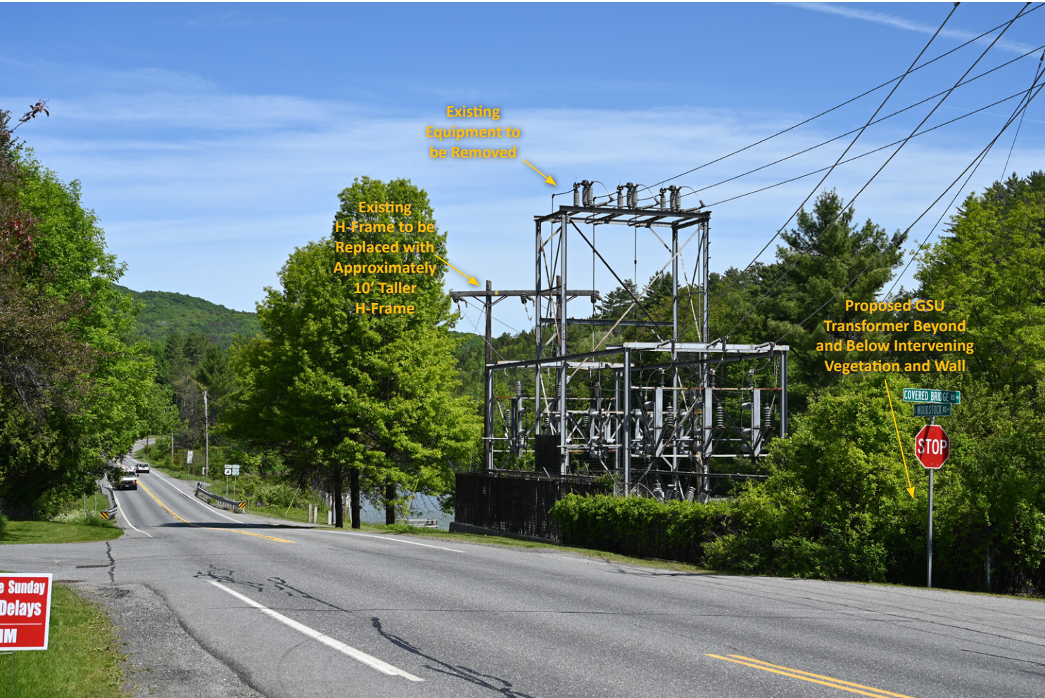
Viewpoint 7: View from Route 4 at the intersection with Butternut Lane, looking northwest towards existing infrastructure to be removed and proposed GSU transformer location (transformer will be below existing wall and out of view). (50mm)
