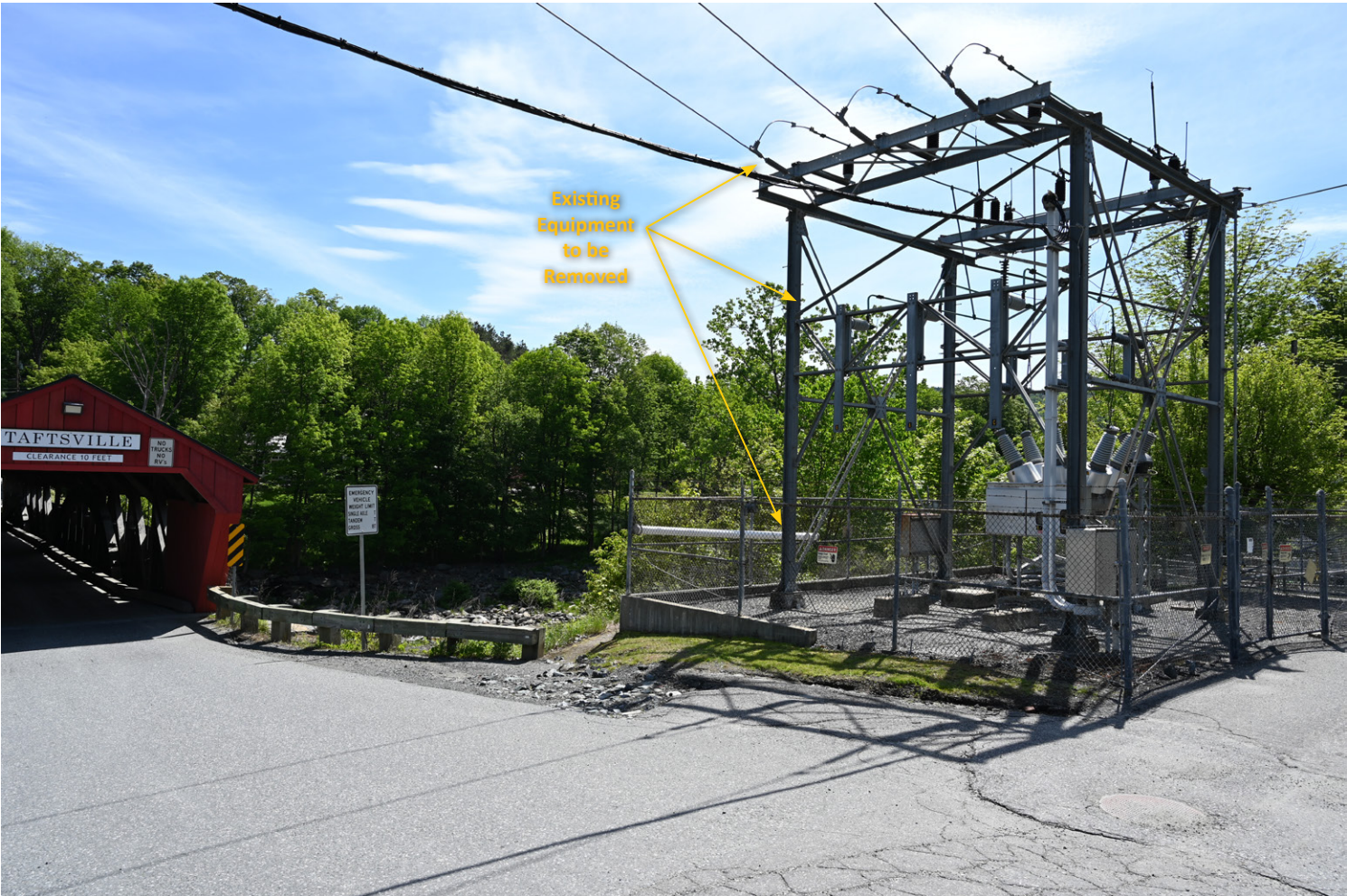
Viewpoint 10: Wide-angle view from the southwest side of the Taftsville Bridge looking east towards existing infrastructure to be removed. (24mm)
