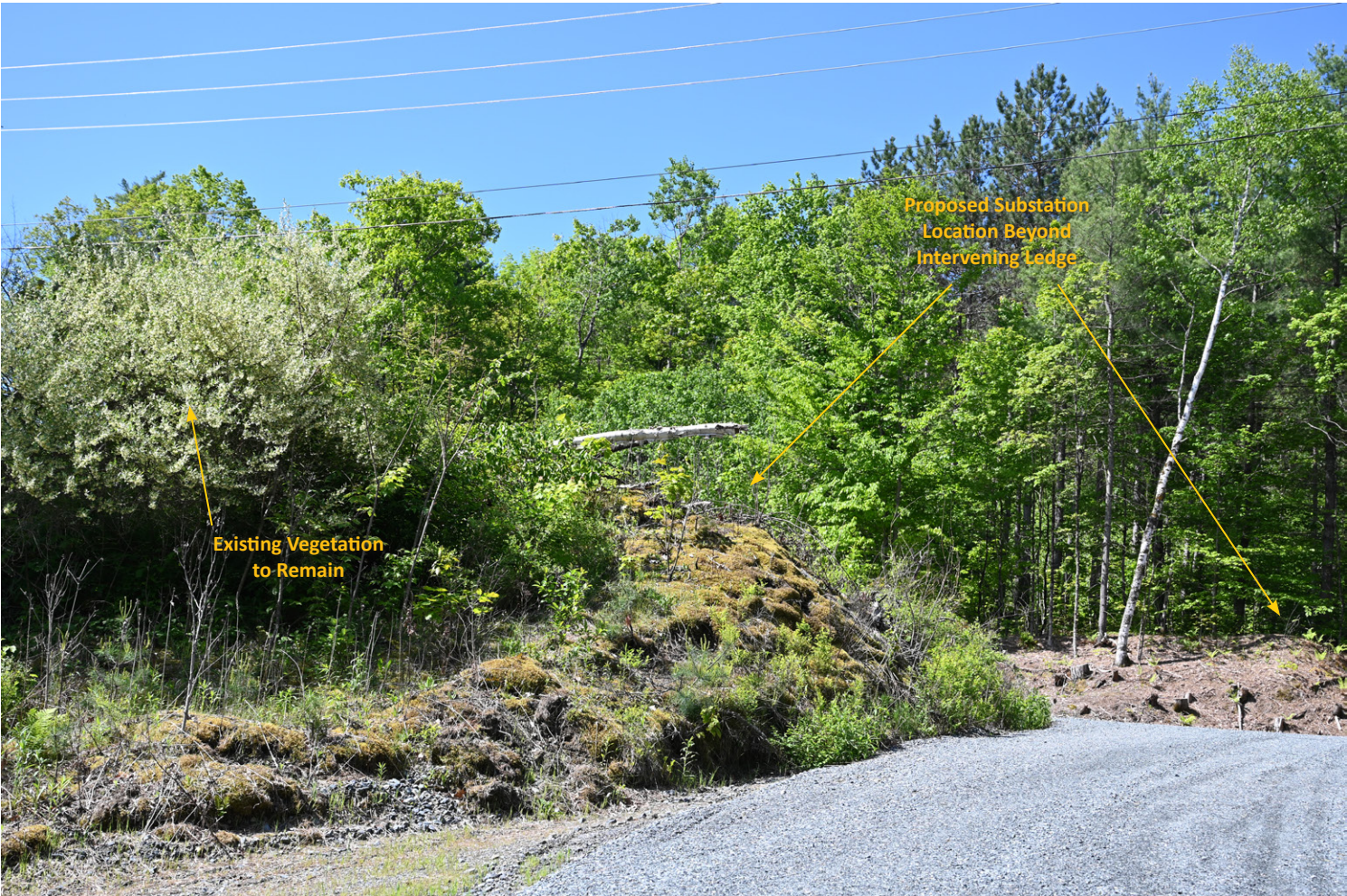
Viewpoint 4: View from existing site gate looking southwest towards the proposed substation location. (50mm)
