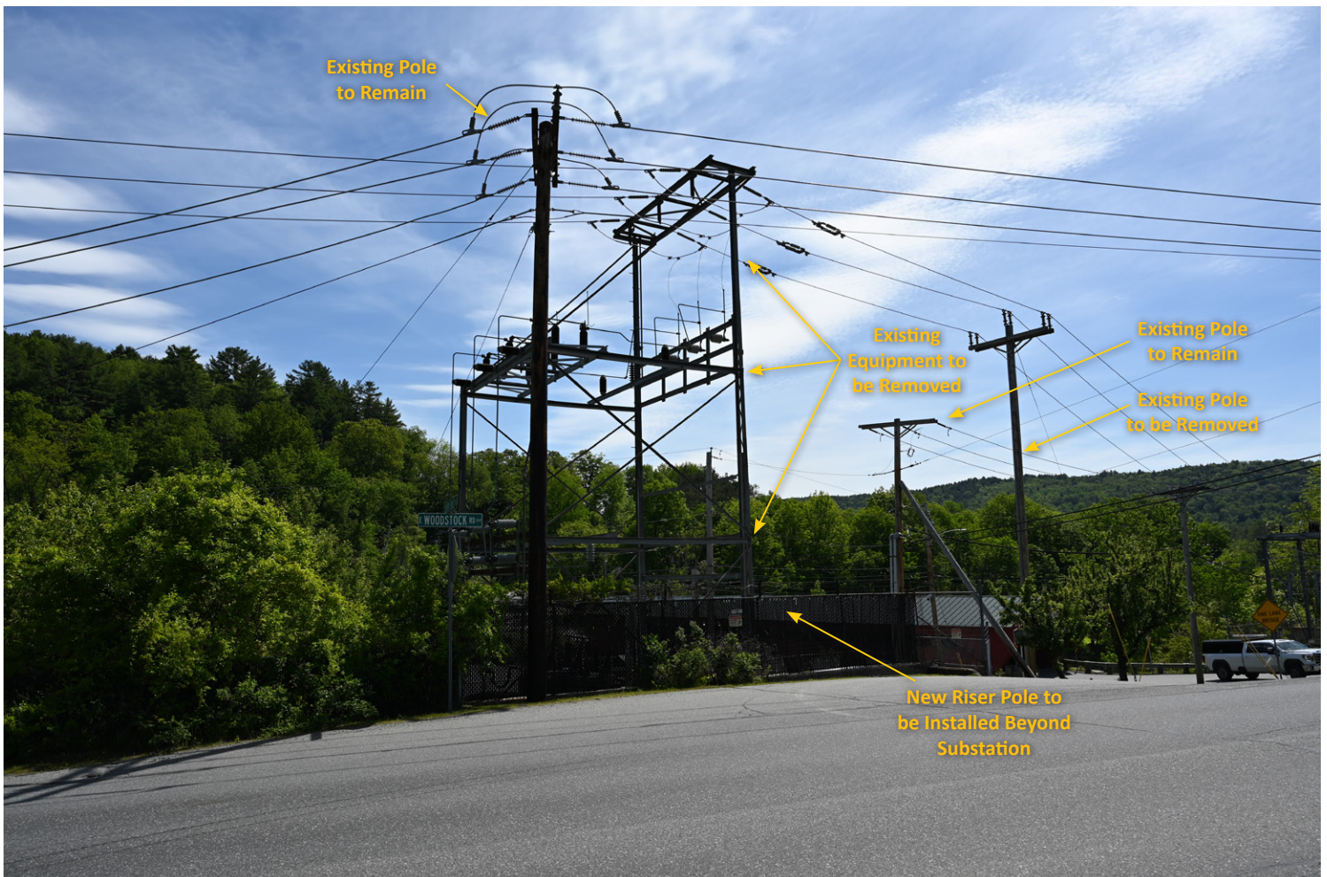
Viewpoint 8: Wide-angle view from Route 4 at the intersection with Happy Valley Road, looking east towards existing infrastructure to be removed. (24mm)
