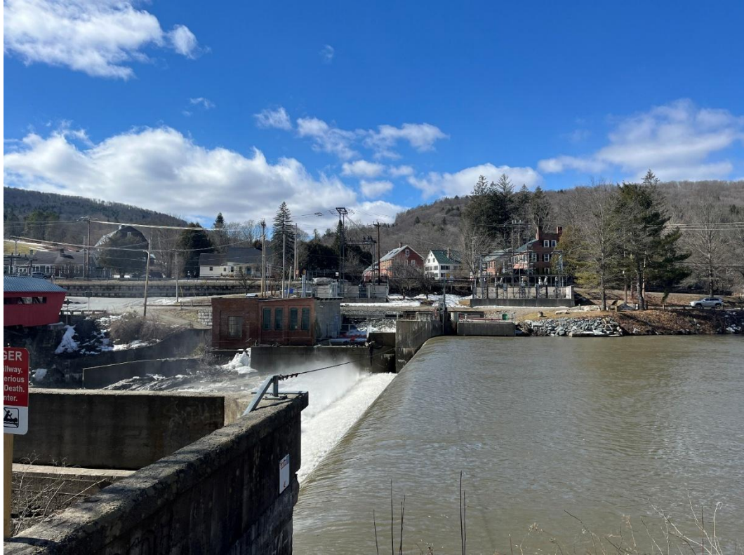
Photograph 22: Taftsville Hydroelectric Station.
