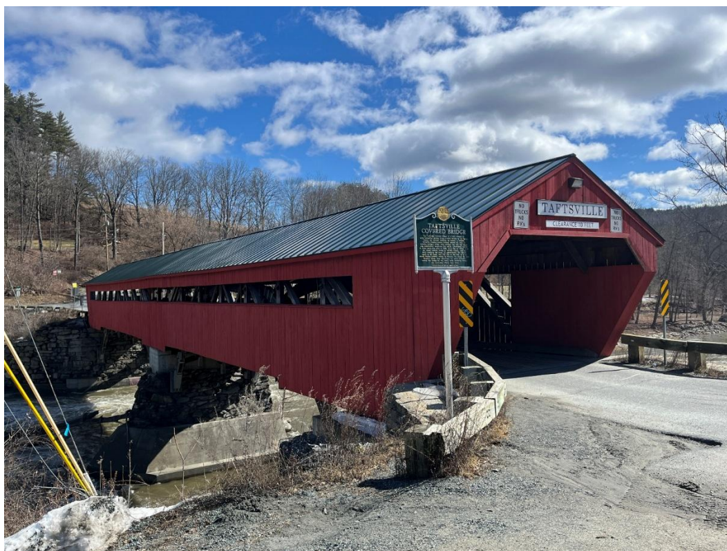
Photograph 20: Taftsville Covered Bridge.
