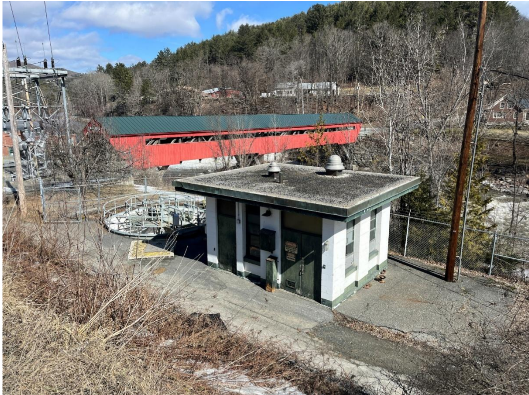
Photograph 19: Water Treatment Plant.
