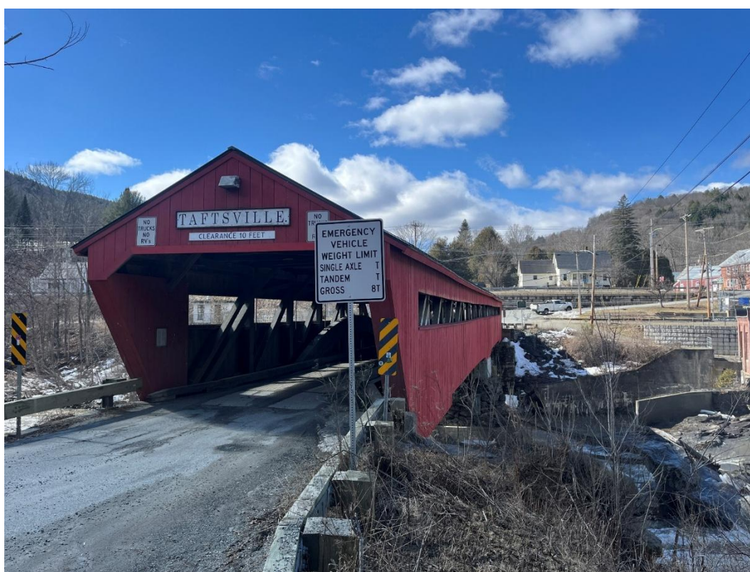
Photograph 21: Taftsville Covered Bridge
