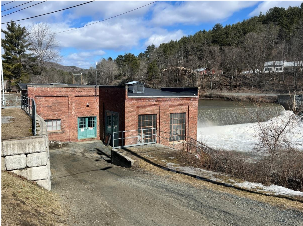
Photograph 23: Taftsville Hydroelectric Station.
