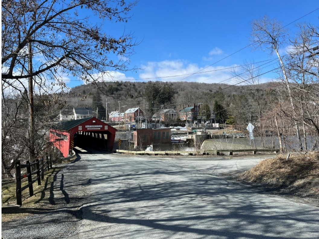
Photograph 1: Looking southwest to the project area from the intersection of Covered Bridge Road and Old River Road (at right).
