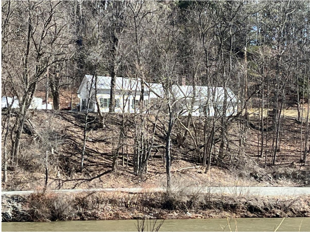
Photograph 28: 87-125 Upper River Road.
