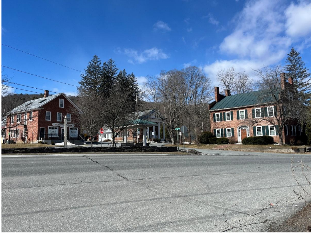
Photograph 10: 2706 US Route 4 / Canopy in small green.
