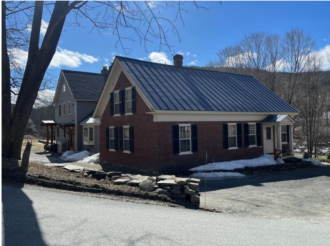
Photograph 27: 201 Covered Bridge Road.
