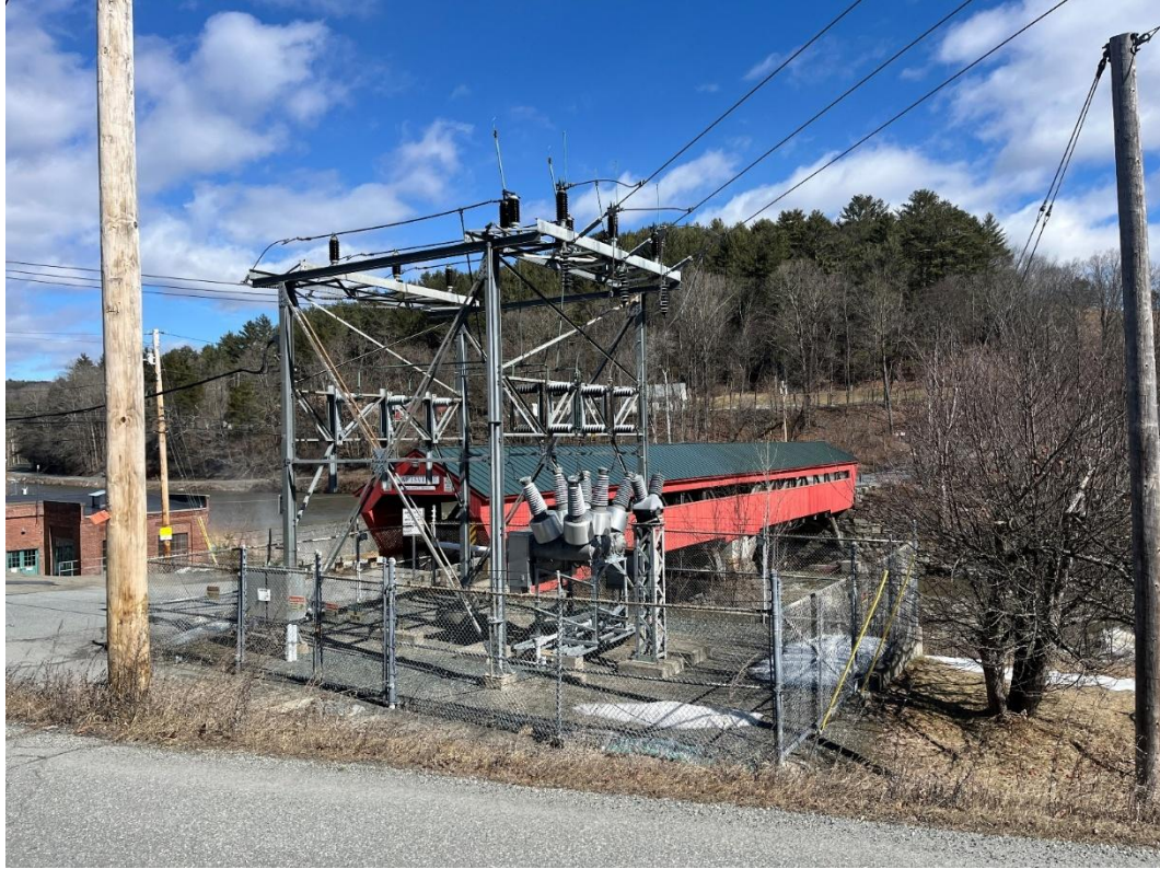
Photograph 4: View looking northeast to the Taftsville Covered Bridge with the hydroelectric station at left and the substation in the foreground.
