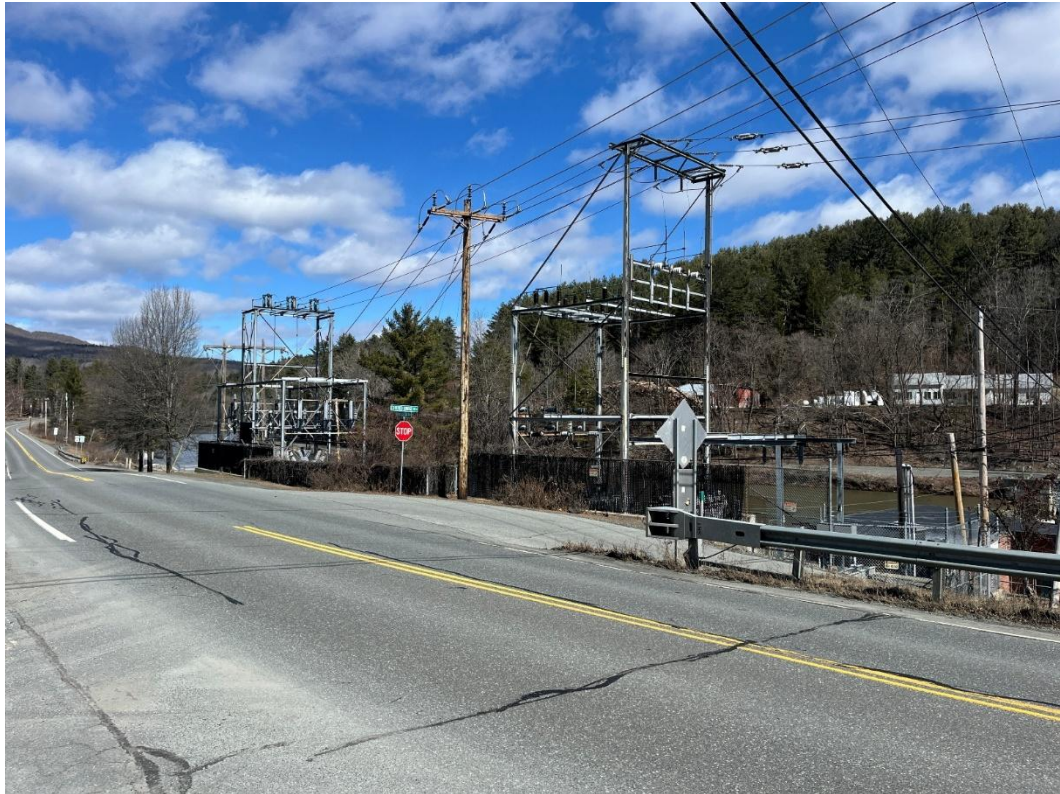
Photograph 3: Looking northeast across US Route 4 to the hydroelectric station.
