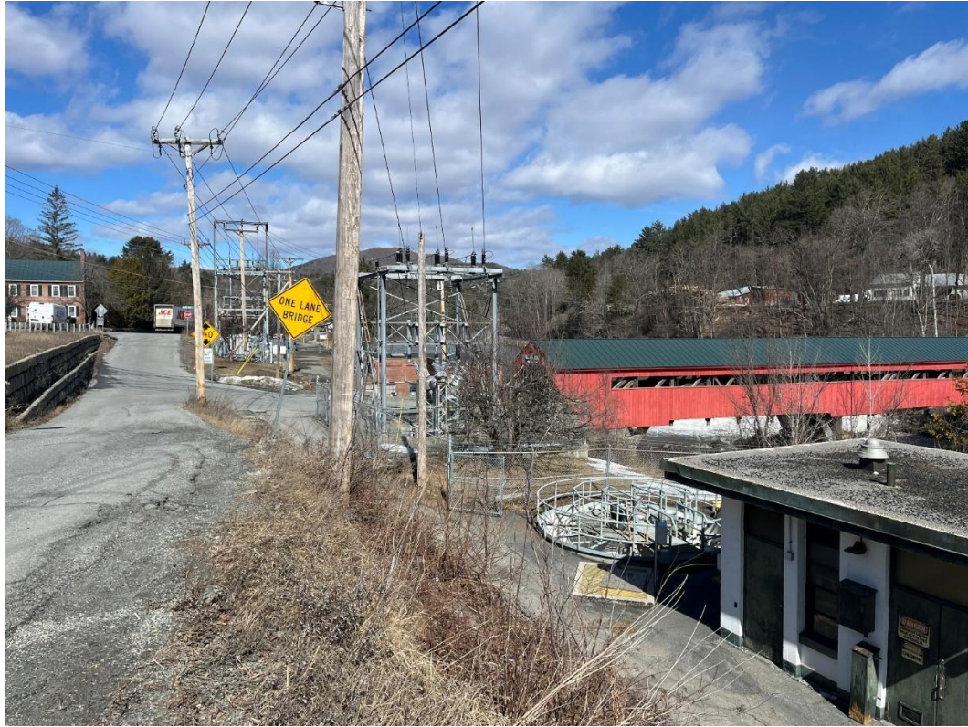
Photograph 2: Looking north/NW to the project area at the substation.
