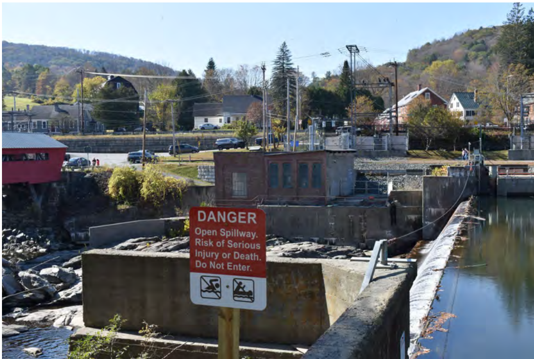
Figure 27. View south of the hydroelectric facility located at the current GMP substation in the North APE of the GMP Taftsville Substation Relocation Project, Woodstock and Hartland, Windsor County, Vermont.
