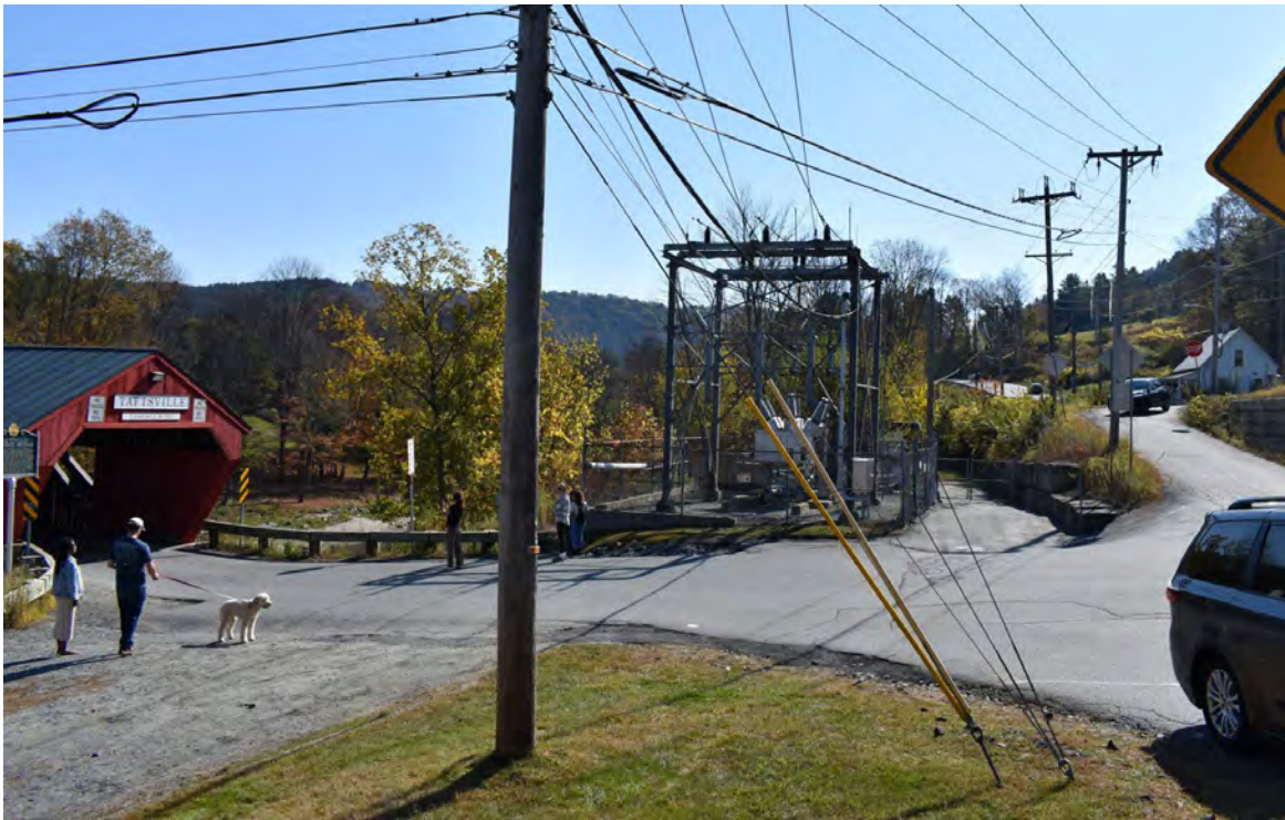
Figure 23. View east of the North Study Area of the GMP Taftsville Substation Relocation Project, Woodstock and Hartland, Windham County, Vermont. Note the current Taftsville Substation in the center midground and the Taftsville Covered Bridge to the left.
