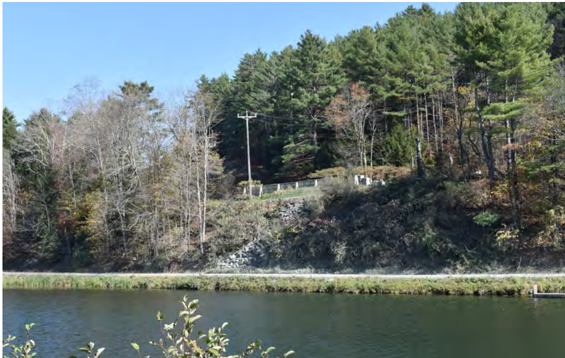
Figure 33. View north showing the riprap reinforced bank between River Road and Upper River Road within the North Study Area of the GMP Taftsville Substation Relocation Project, Woodstock and Hartland, Windsor County, Vermont.
