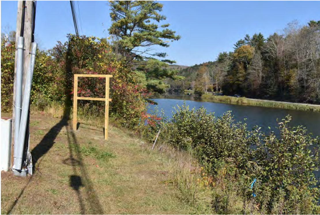
Figure 32. View west showing a utility pole and indications of buried electrical conductors within the North Study Area of the GMP Taftsville Substation Relocation Project, Woodstock and Hartland, Windsor County, Vermont.
