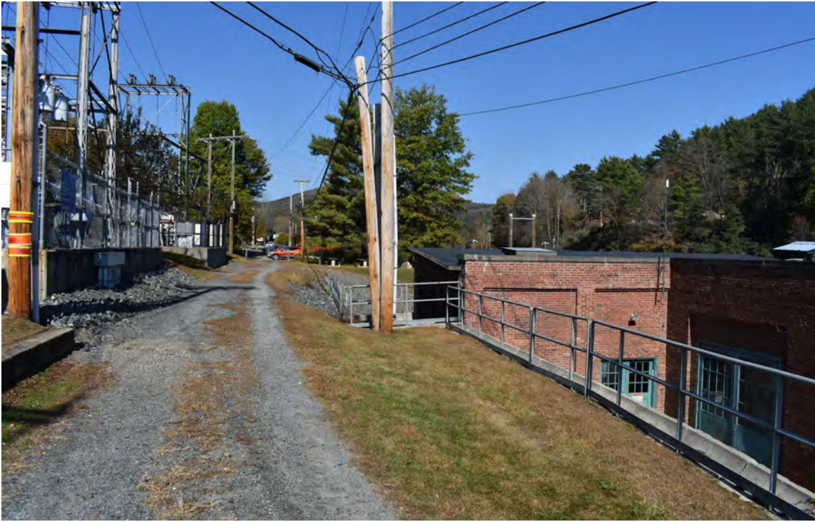
Figure 22. View west of the North Study Area of the GMP Taftsville Substation Relocation Project, Woodstock and Hartland, Windham County, Vermont. Note the current Taftsville Substation structures to the left of the photo.
