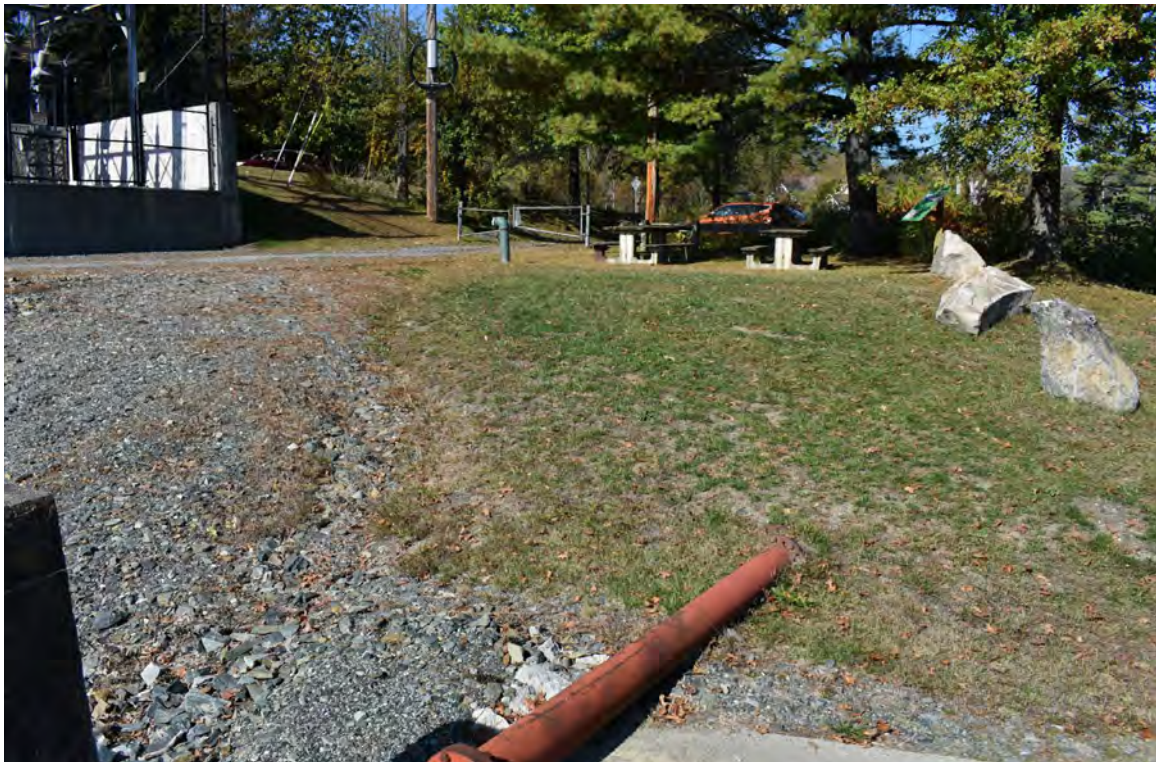
Figure 31. View southwest showing a buried pipeline within the North Study Area of the GMP Taftsville Substation Relocation Project, Woodstock and Hartland, Windsor County, Vermont.
