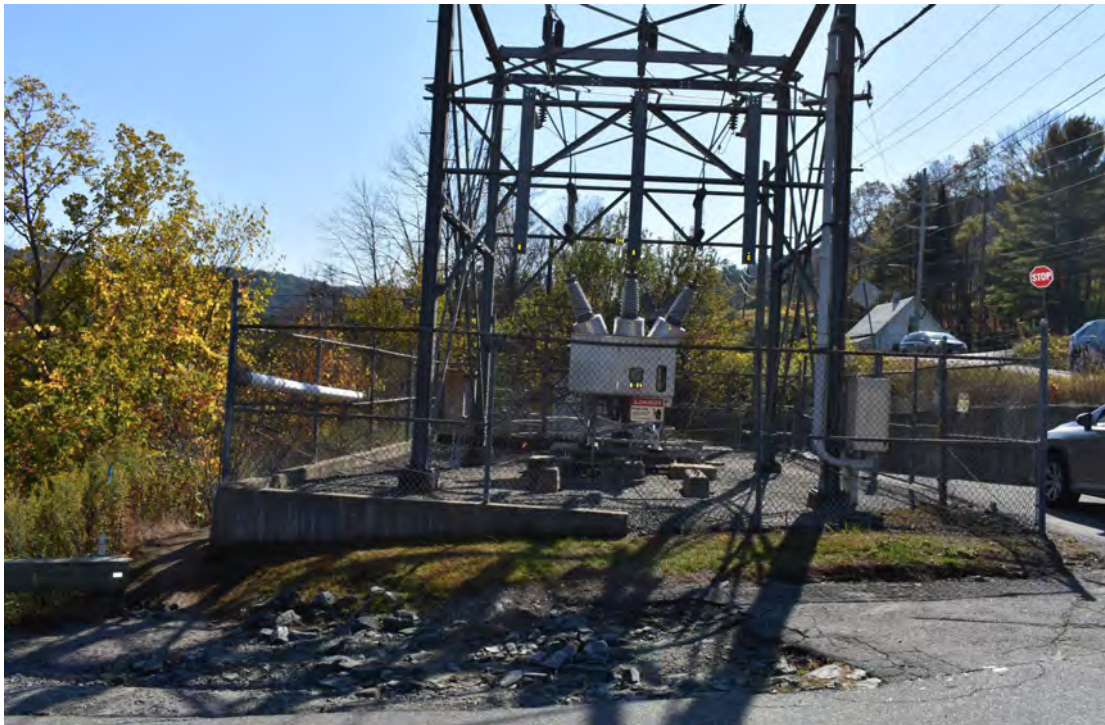
Figure 24. View east of the Transmission East substation structure of the Taftsville Substation, located in the North Study Area of the GMP Taftsville Substation Relocation Project, Woodstock and Hartland, Windham County, Vermont.
