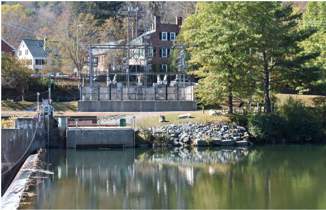
Figure 30. View south of the small section of retaining wall which may be related to the former Taft scythe factory located within the North Study Area of the GMP Taftsville Substation Relocation Project, Woodstock and Hartland, Windsor County, Vermont.
