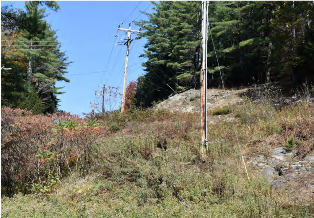
Figure 34. View north up the transmission line corridor within the North Study Area of the GMP Taftsville Substation Relocation Project, Woodstock and Hartland, Windsor County, Vermont. Note the steep slope and rocky terrain.
