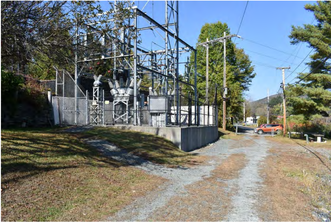
Figure 26. View west of the Distribution substation structure of the Taftsville Substation, located in the North Study Area of the GMP Taftsville Substation Relocation Project, Woodstock and Hartland, Windham County, Vermont.
