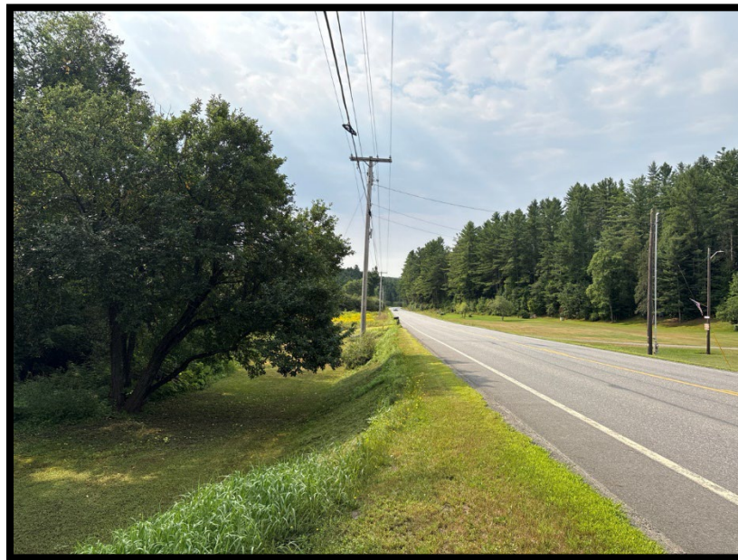
Utility corridor along Route 14 (8/10/26)
