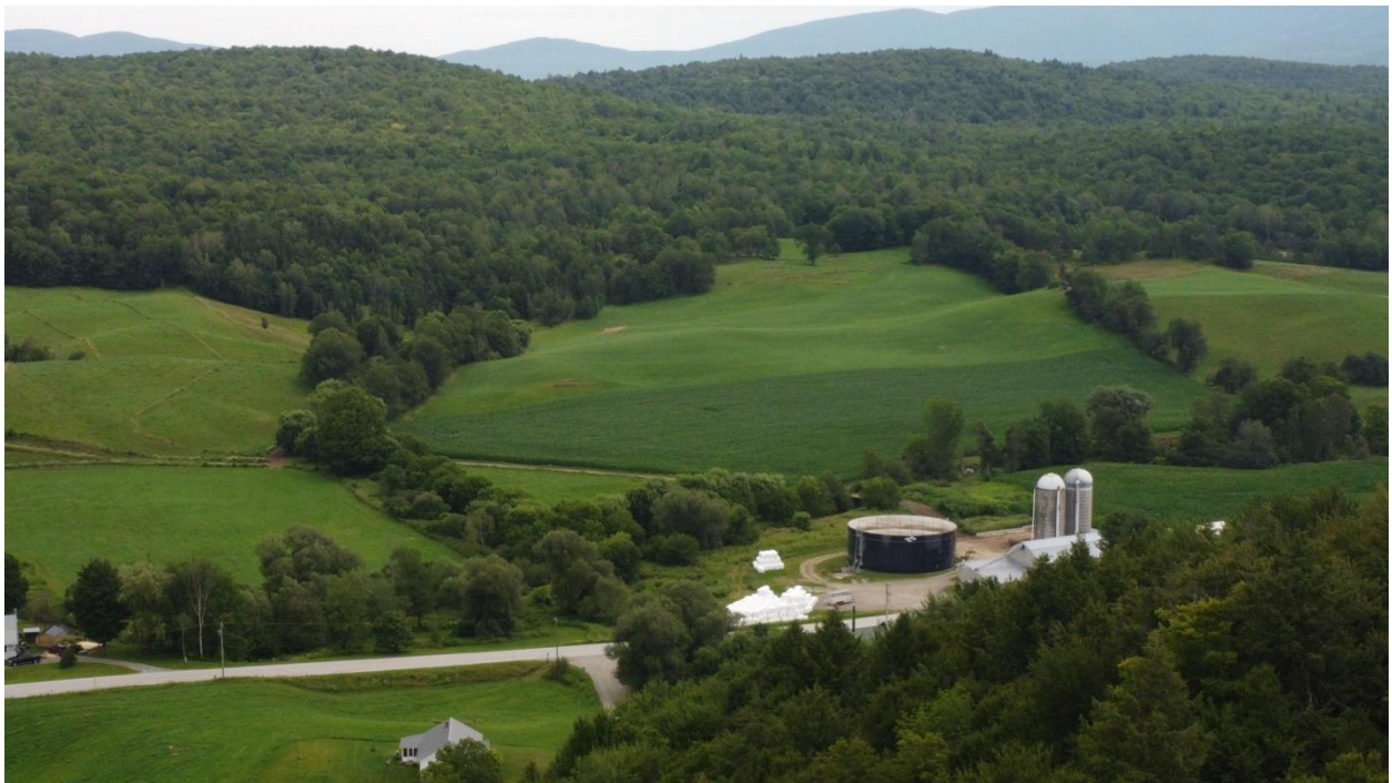
Southeast view from top of proposed tower.
