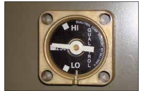
Figure 5. Liquid level gauge.
