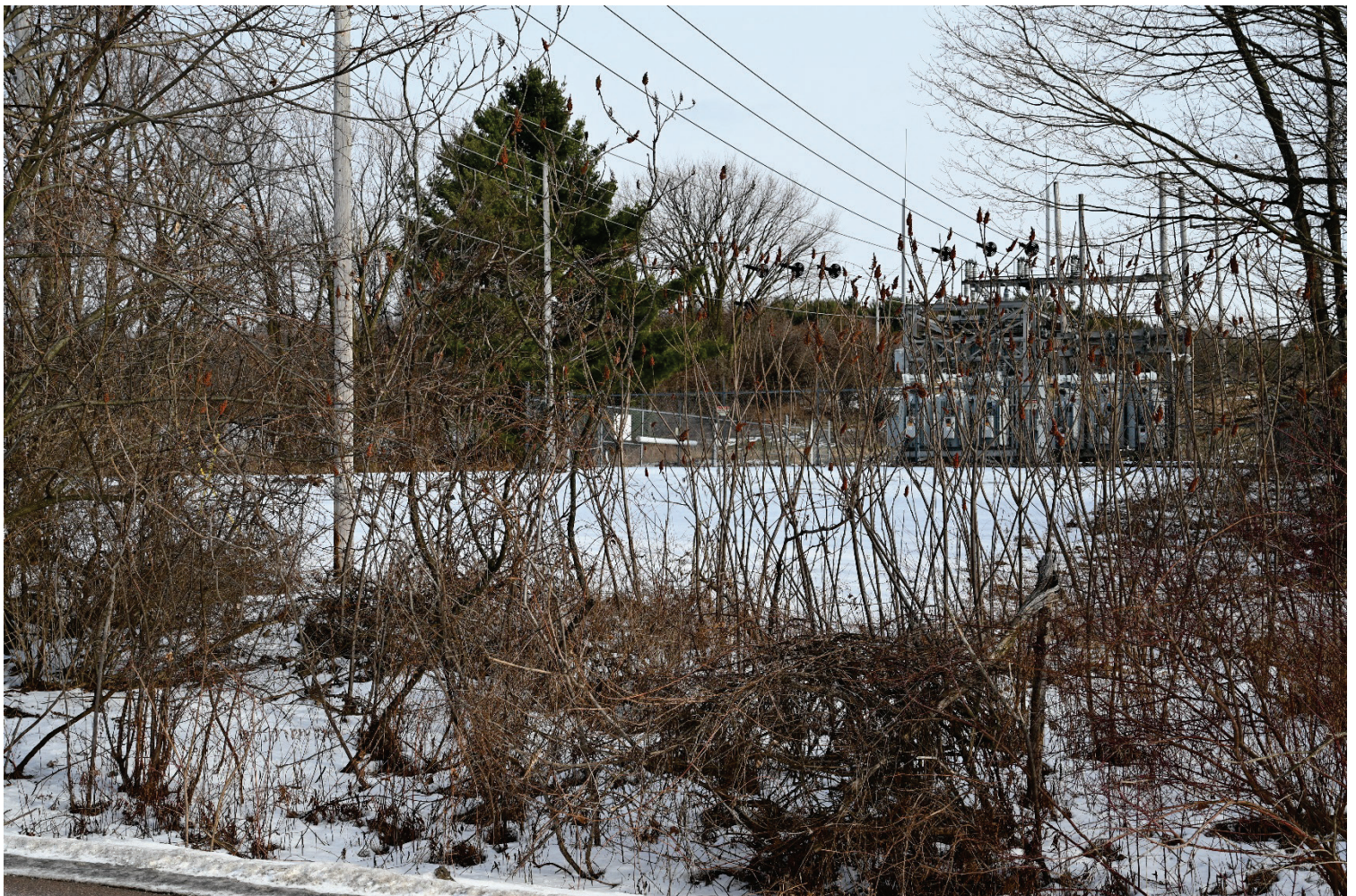
Viewpoint 7: View from Ballard Road looking east towards the existing substation. (50mm)
