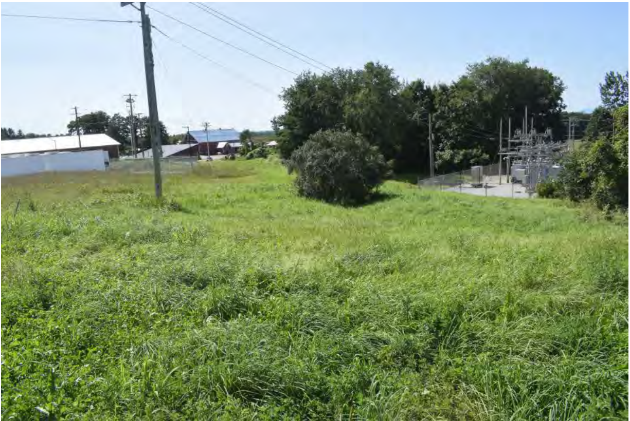
Figure 20. View southwest of the existing Green Mountain Power Georgia Substation Upgrade Project, Franklin County, Vermont. Note gradual slope west towards substation. Also note the newly constructed BESS facility to the left of the image.
