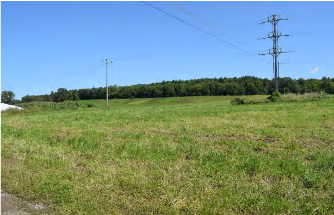
Figure 18. View northeast showing the transmission line running east of the existing Green Mountain Power Georgia Substation Upgrade Project, Franklin County, Vermont.
