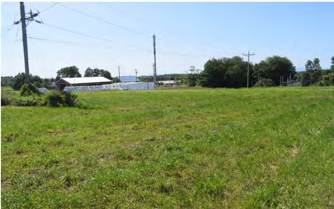
Figure 19. View southwest from the level landform looking toward the existing Green Mountain Power Georgia Substation Upgrade Project, Franklin County, Vermont. Note elevation difference between field and substation. Also note the newly constructed BESS facility to the center left of the image.
