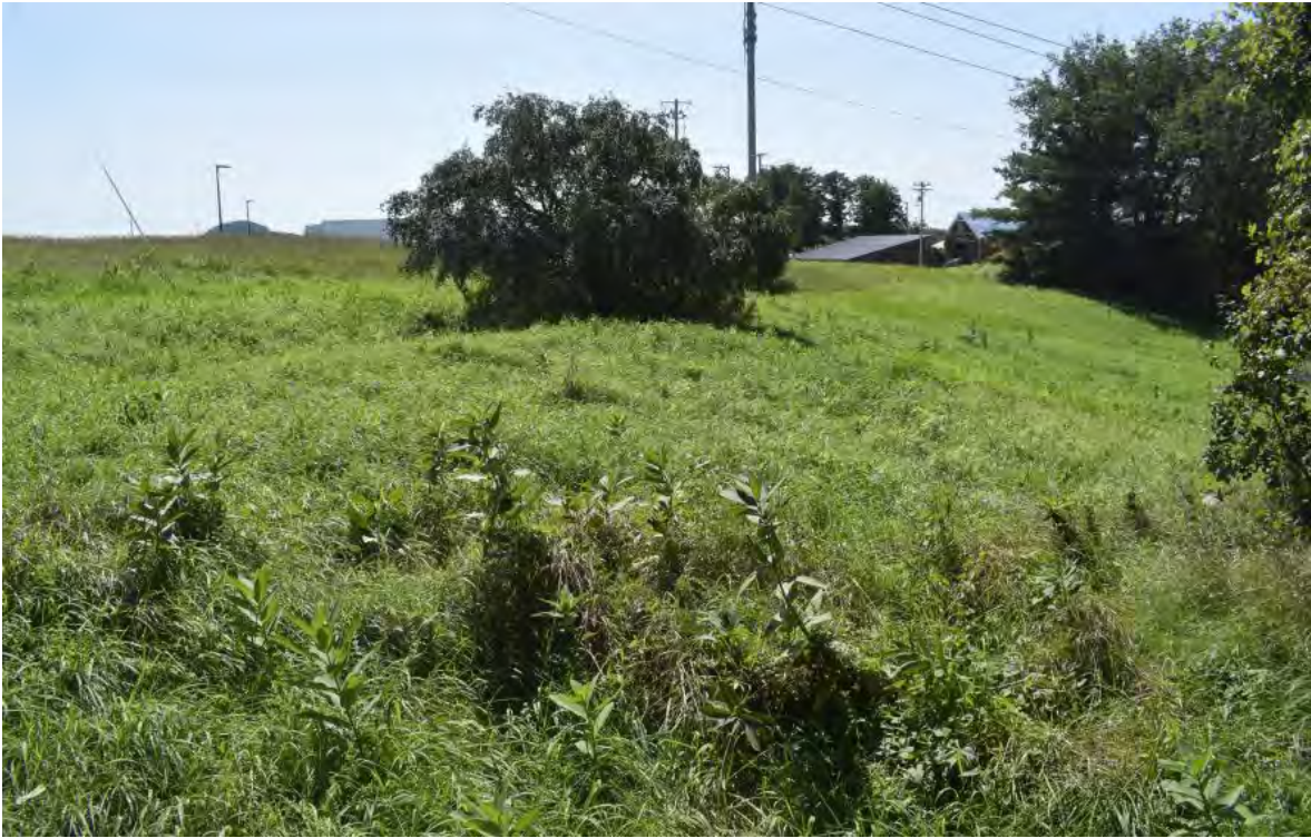
Figure 16. View south of transmission line running east of existing Green Mountain Power Georgia Substation Upgrade Project, Franklin County, Vermont.
