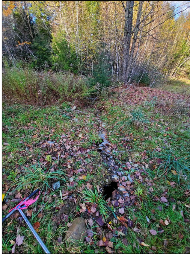
Photograph 5: View of culvert between Wetlands B and C with Wetland C in the background, view looking north.
