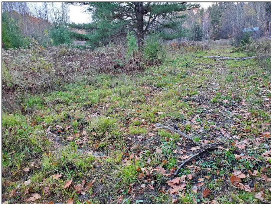
Photograph 6: View of culvert between Wetlands B and C with Wetland B on left side of photograph and cabin in the background, view looking west.
