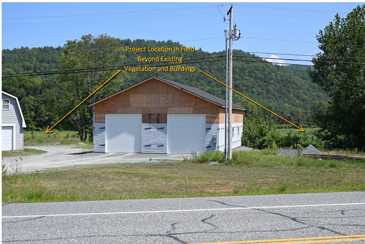
Viewpoint 6: View from Vermont Route 103 looking east towards the Project site. (50mm)
