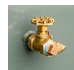
Drain Sample Valve
