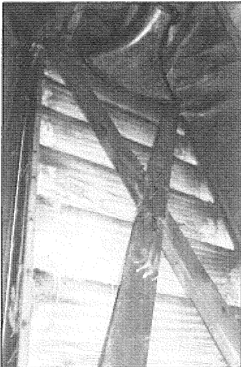
32. Belfry level, detail of louvers and screening
