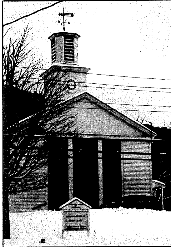
4. Front façade, looking west
