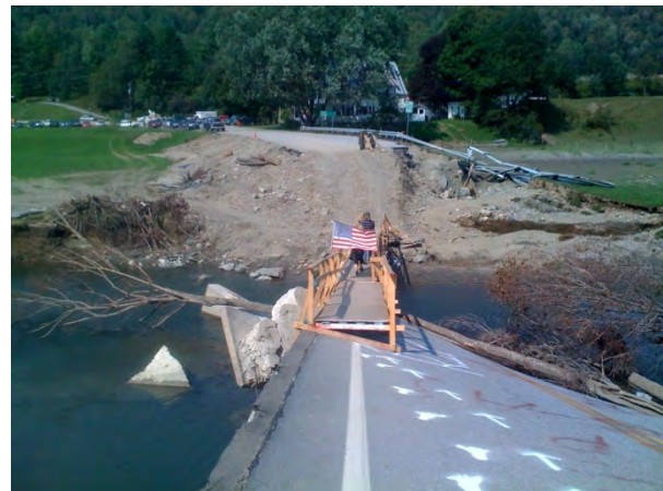
6 - Temporary footbridge over White River (Source: VTrans)
