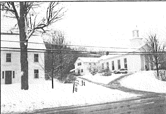
38. Looking northwest at Federated Church (#1) With #2 on left.
