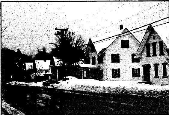
40. South Main St. along west side of green, looking south (#5 on right).
