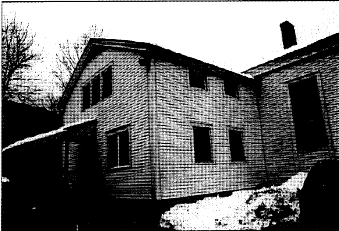
9. Rear ell, view looking northwest
