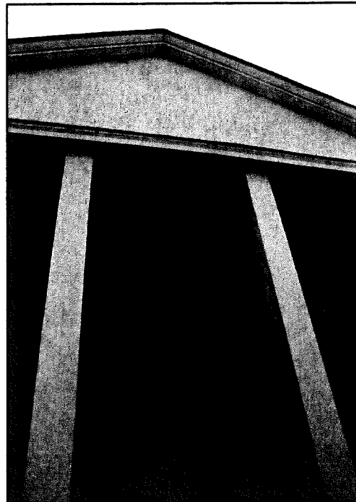
6. Front entry detail, looking west
