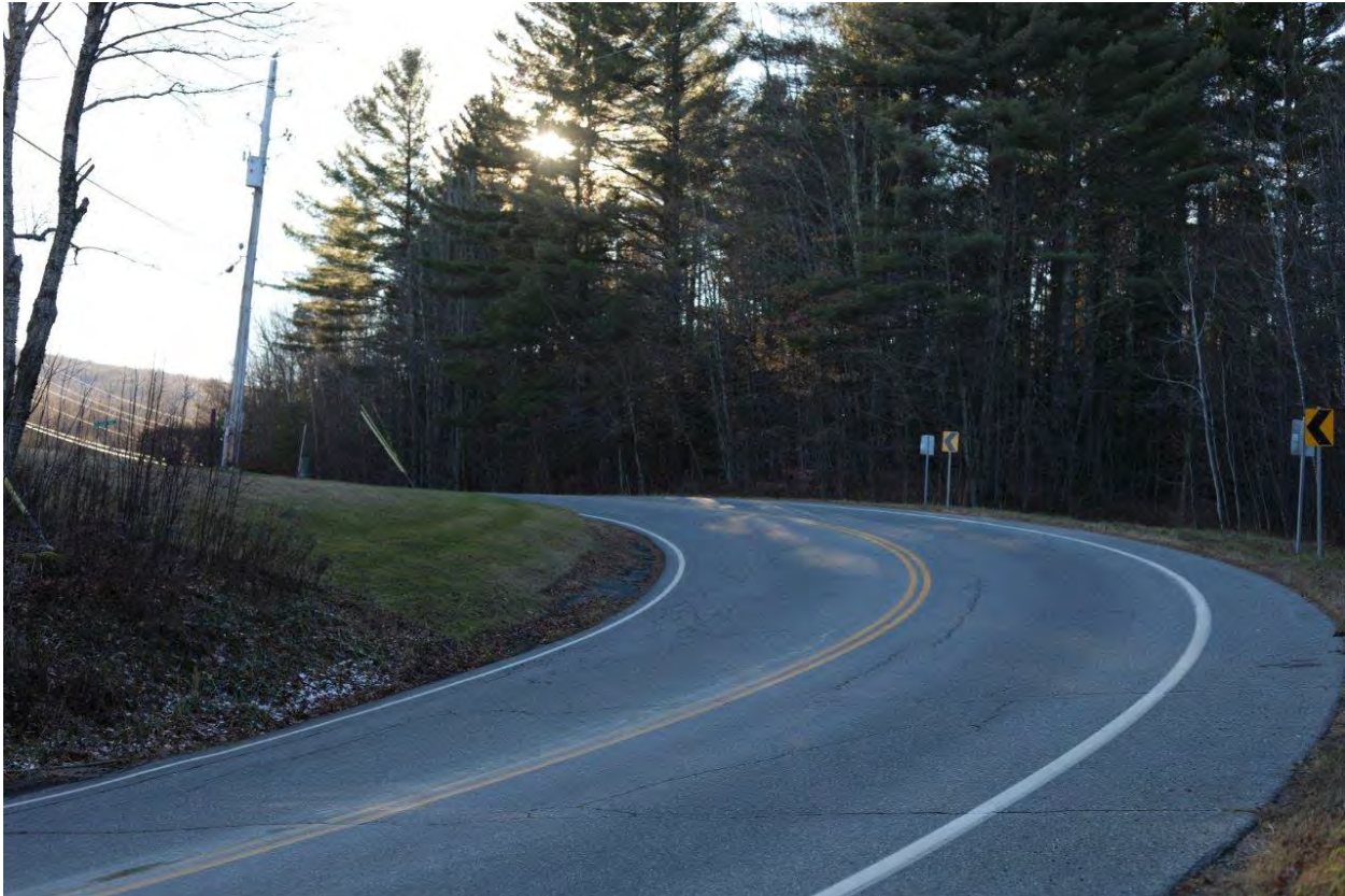
Photo 1: View from VT Route 242 approximately 500' north of project entrance looking southwesterly.
