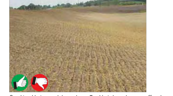
Good tracking up and down slope. Tracking slows down runoff and promotes infiltration. More mulch is needed.
