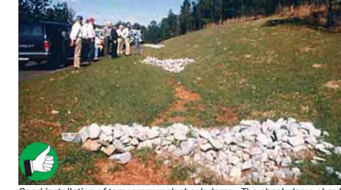
Good installation of temporary rock check dams. The check dams should extend up the sides of the banks. Middle section should be lower than the sides. Clean out sediment as it accumulates. Remove check dams after site and channel are stabilized with vegetation.
