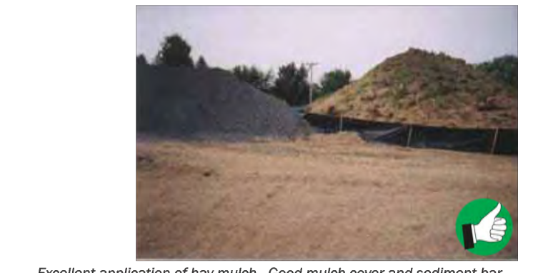
Excellent application of hay mulch. Good mulch cover and sediment barrier around soil stockpile.
