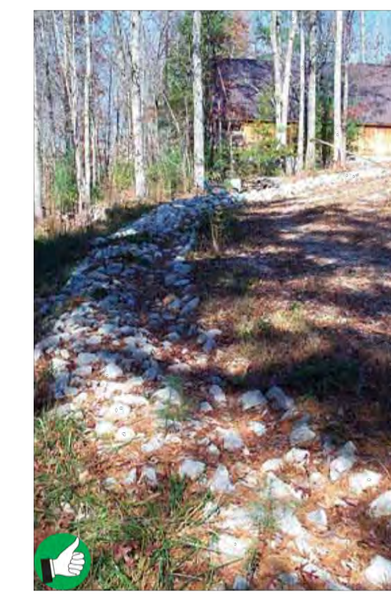
Good installation of rock-lined berm to divert rain runoff around residential construction site on steep slope near a river. Diversion ditches can be lined with grass if channel slopes are 5% or less, and with 4 inch stone if they are steeper.
