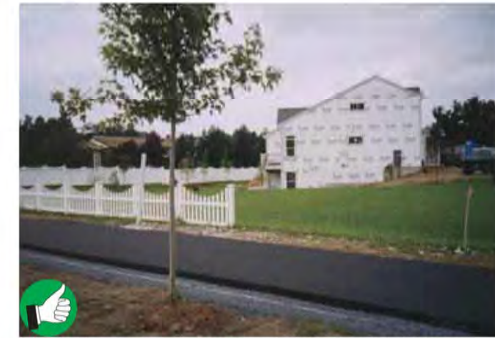
Lawn is fully established before construction is completed at this home site.
