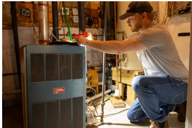
A VGS Building Analyst evaluating an aging heating system to help support the upgrade to high-efficiency equipment.
