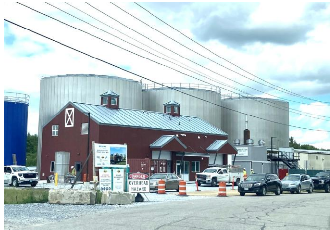
Industrial site showcasing high-performance design principles that support efficient operations and reduced energy use.
