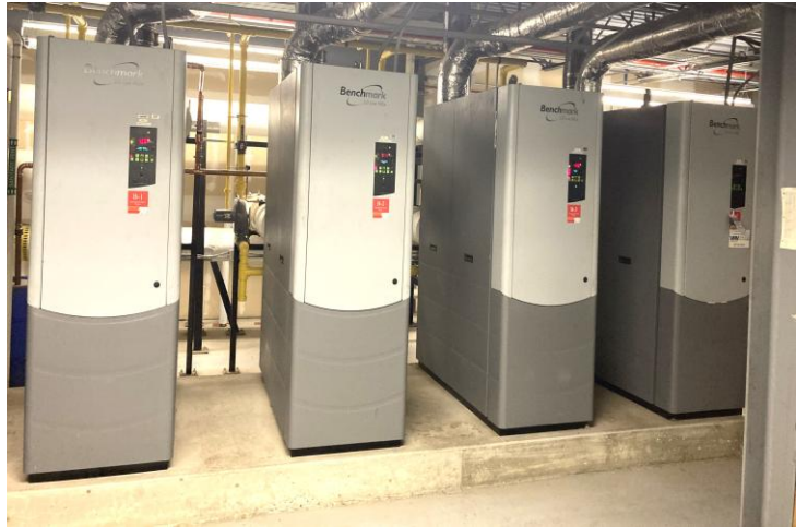
Advanced condensing boiler system providing efficient, cost-effective heating and hot water for commercial operations.
