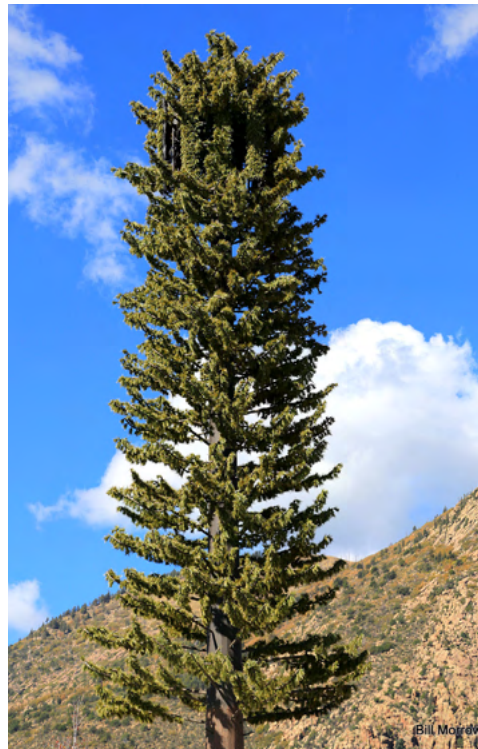
An example of a Cell Tower in Disguise | © Bill Morrow
