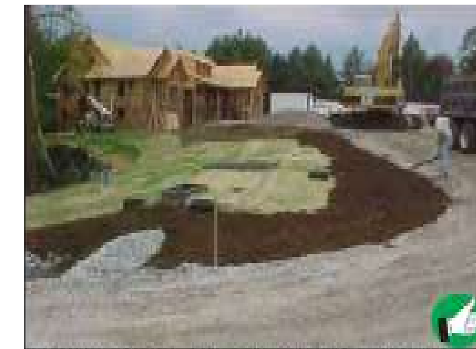
Within 48 hours of final grading, erosion control matting and mulch have been applied.
