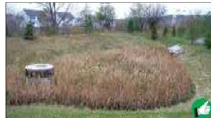
Install all permanent stormwater treatment practices before commencing any impervious surfaces on site. This stormwater wetland treats stormwater runoff from the adjacent parking lot. 24
