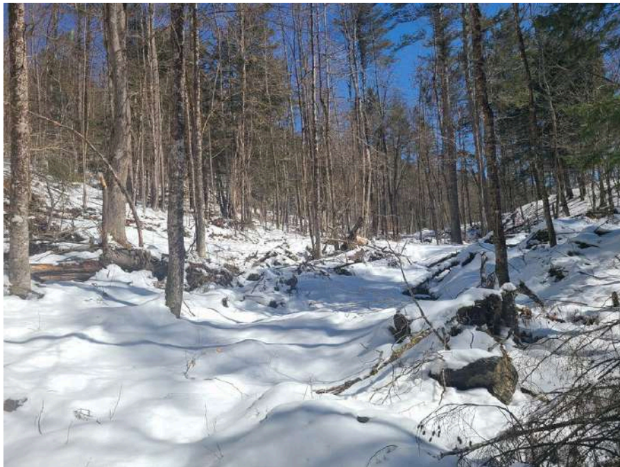
6. View along a portion of the proposed access easement and overhead utilities.
