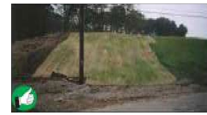
Excellent stabilization of large slopes to limit the area of disturbance. Make sure to install erosion control matting within 48 hours of grading to ensure good contact between soil and mat. 27
