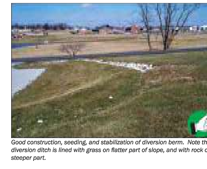
Good construction, seeding, and stabilization of diversion berm. Note that diversion ditch is lined with grass on flatter part of slope, and with rock on steeper part. 17
