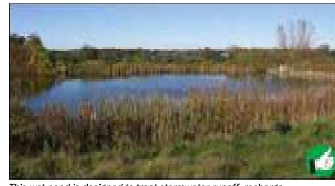
This wet pond is designed to treat stormwater runoff, recharge groundwater, regulate the flow of water into nearby streams, and prevent downstream flooding. 24
