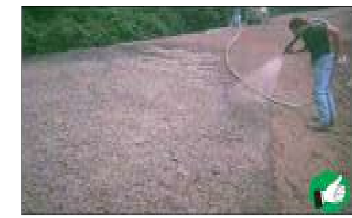
Hydroseeding exposed soil is a good option for stabilizing large areas. Hydroseed is a mixture of seed, fertilizer, water and a tackifier to hold the seed in place before it germinates. 28
