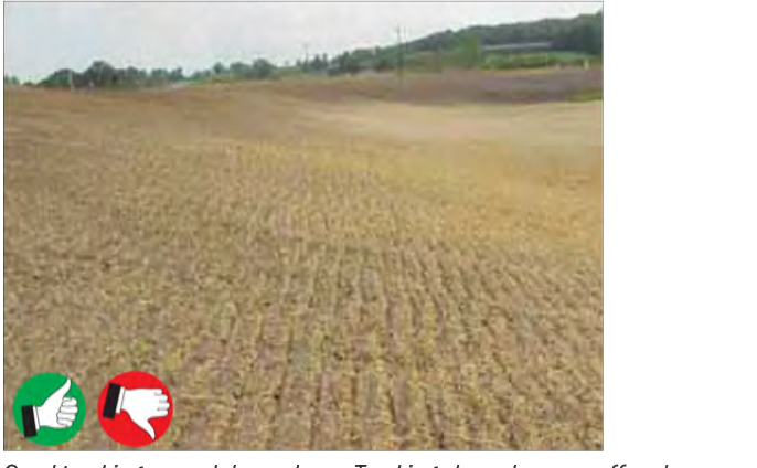
Good tracking up and down slope. Tracking slows down runoff and promotes infiltration. More mulch is needed. Stabilize Exposed Soil 27
