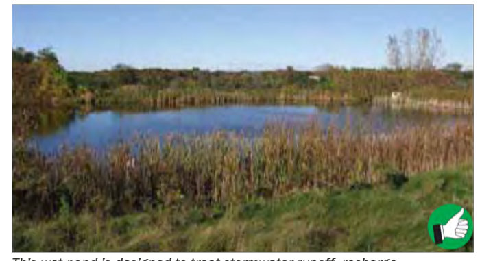
This wet pond is designed to treat stormwater runoff, recharge groundwater, regulate the flow of water into nearby streams, and prevent downstream flooding. 24
