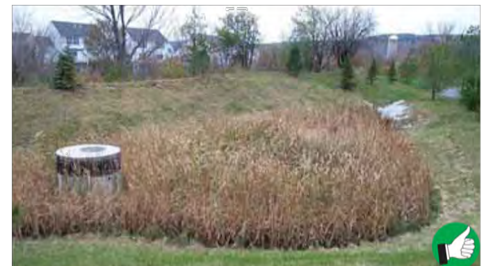
Install all permanent stormwater treatment practices before constructing any impervious surfaces on site. This stormwater wetland treats stormwater runoff from the adjacent parking lot. Construct Permanent Controls 24
