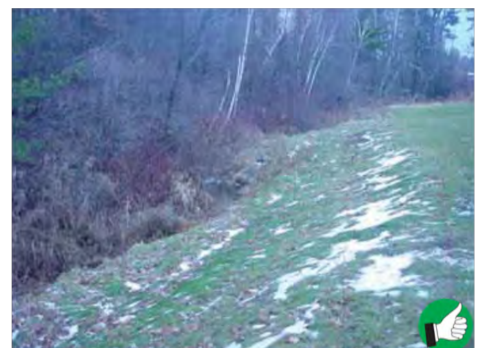
Stabilization and seeding of slopes before winter will reduce or eliminate erosion in the spring. The grass on this slope is holding the soil in place and promoting infiltration of the melting snow. 30
