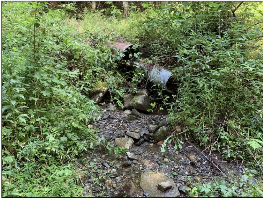
Culvert below existing logging road; intermittent stream
