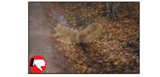
Hay bales must not be used as check dams due to their high failure rates.
