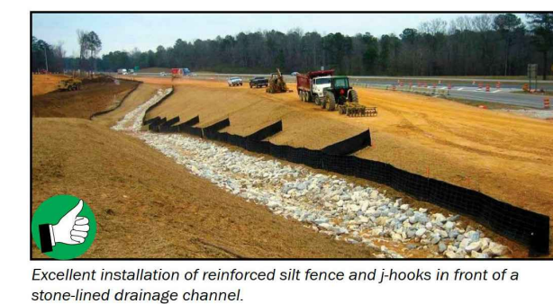
Excellent installation of reinforced silt fence and jhooks in front of a stone-lined drainage channel.
