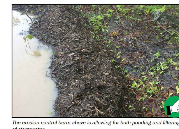
The erosion control berm above is allowing for both ponding and filtering of stormwater.
