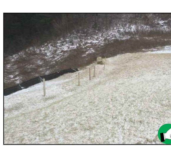
Stabilization and seeding of slopes before winter will reduce or eliminate erosion in the spring.
