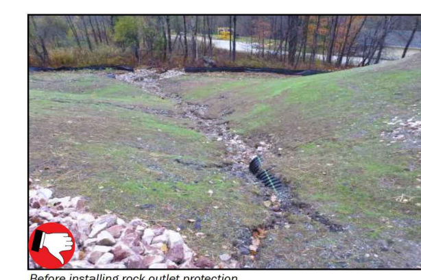
Before installing rock outlet protection
