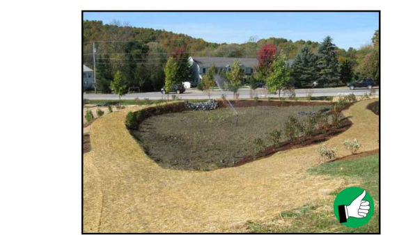
Infiltrating stormwater practices such as this bioretention system should be kept offline until the drainage area has been fully stabilized.
