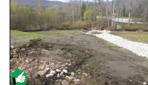
After installing rock outlet protection
