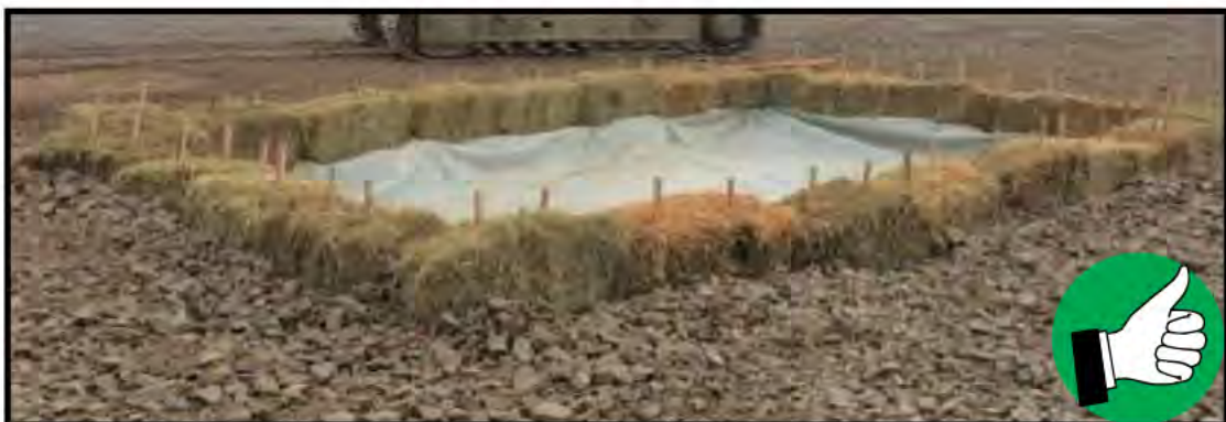
ABOVE GRADE STRAW BALE CONCRETE WASHOUT DETAIL
