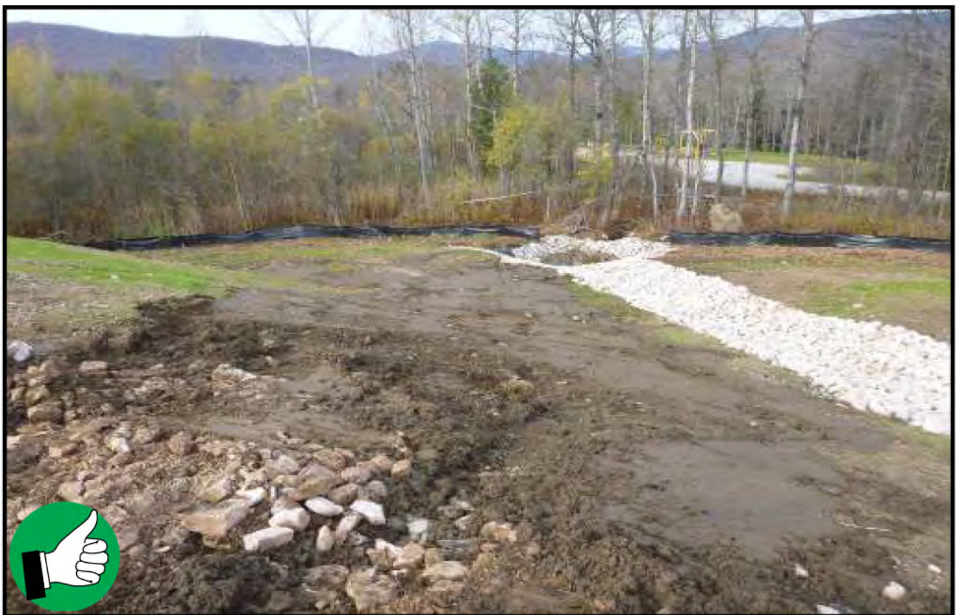
After installing rock outlet protection
