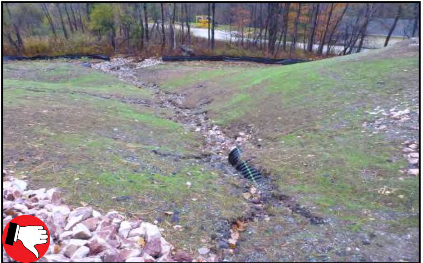
Before installing rock outlet protection
