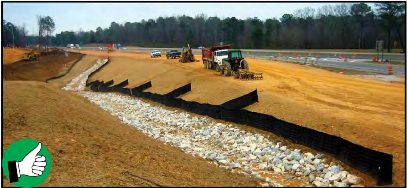
Excellent installation of reinforced silt fence and j-hooks in front of a stone-lined drainage channel.
