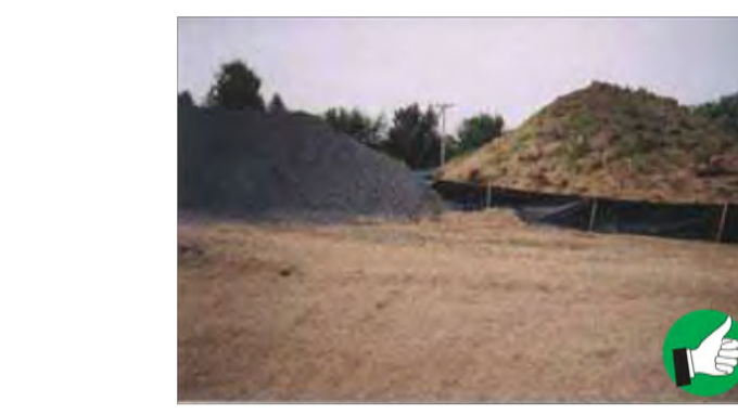
Excellent application of hay mulch. Good mulch cover and sediment barrier around soil stockpile.
