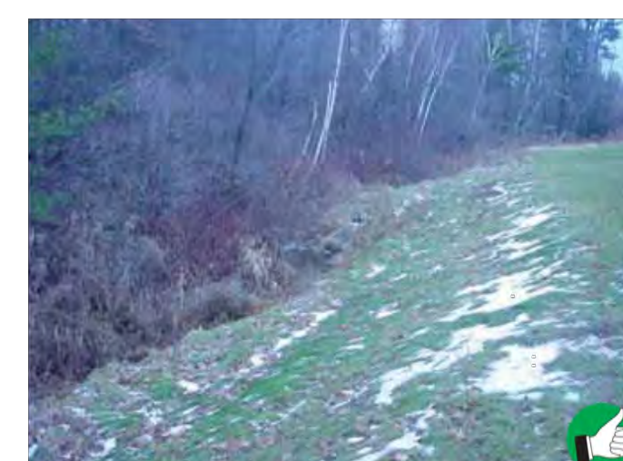
Stabilization and seeding of slopes before winter will reduce or eliminate erosion in the spring. The grass on this slope is holding the soil in place and promoting infiltration of the melting snow.
