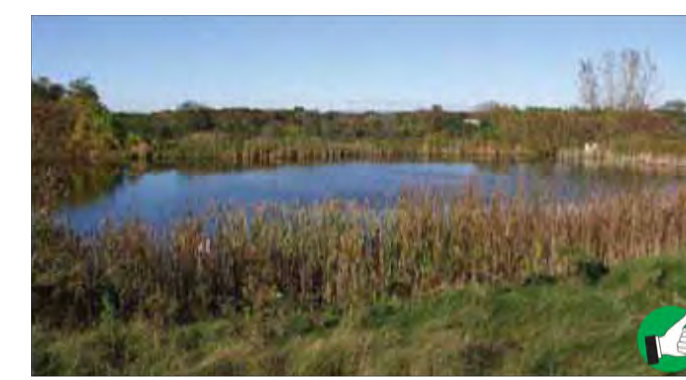
This wet pond is designed to treat stormwater runoff, recharge groundwater, regulate the flow of water into nearby streams, and prevent downstream flooding.
