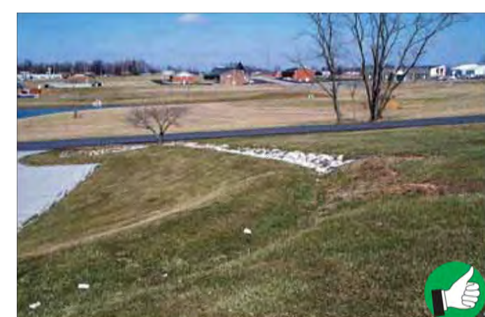
Well built vegetated berm diverting runoff. Diversion berms and ditches should be seeded after construction. Use matting if slopes are steep.
