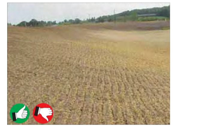
Good tracking up and down slope. Tracking slows down runoff and promotes infiltration. More mulch is needed.
