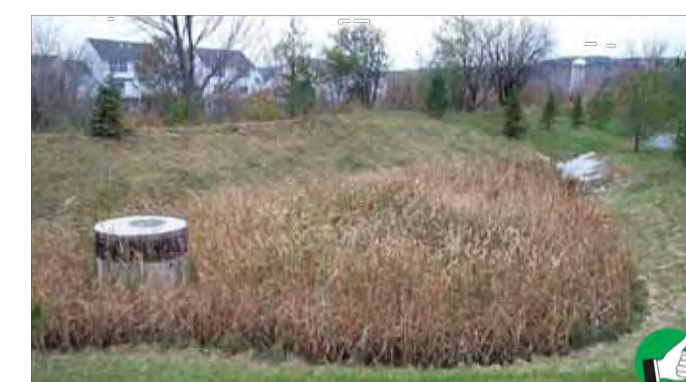
Install all permanent stormwater treatment practices before constructing any impervious surfaces on site. This stormwater wetland treats stormwater runoff from the adjacent parking lot.
