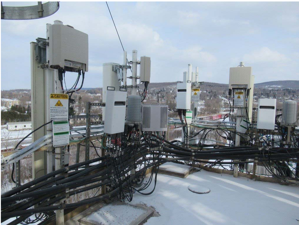
Photo 4: Sample photo illustrating the existing steel frames.
