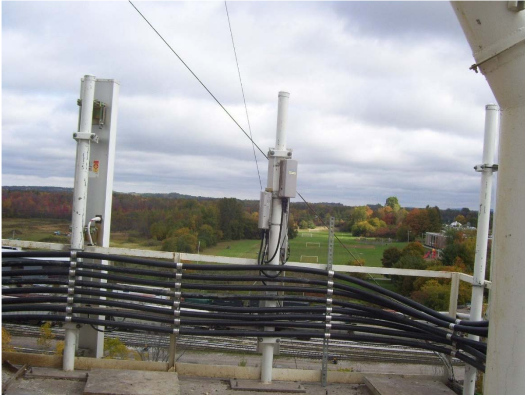
Photo 5: Sample photo illustrating the existing steel frames.
