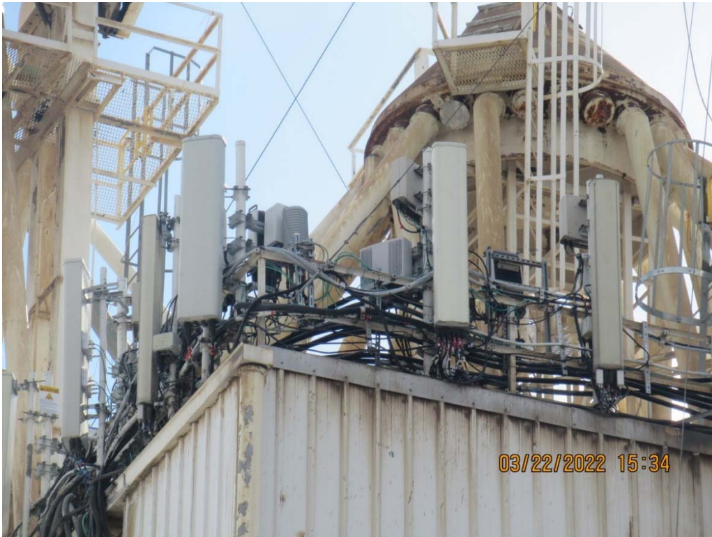
Photo 1: Sample photo illustrating the existing Alpha sector antennas and RRH's.
