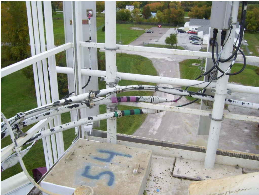
Photo 6: Sample photo illustrating the existing steel frames.
