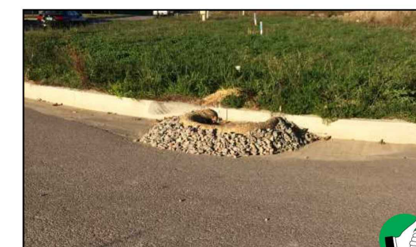
Use of stone inlet protection with the incorporation of a straw wattle in place of cinder blocks for the stone and block specification.
