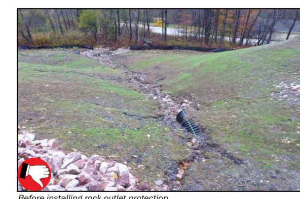
Before installing rock outlet protection
