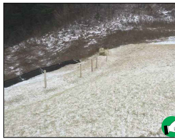
Stabilization and seeding of slopes before winter will reduce or eliminate erosion in the spring.
