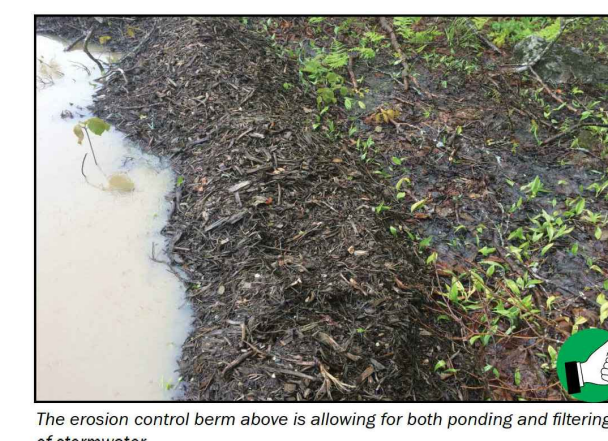
The erosion control berm above is allowing for both ponding and filtering of stormwater.
