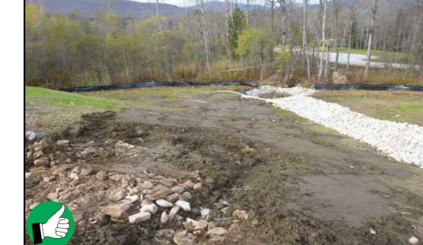
After installing rock outlet protection
