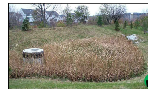
Install all permanent stormwater treatment practices before constructing any impervious surfaces on site. This stormwater wetland treats stormwater runoff from the adjacent parking lot.
