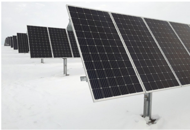
Figure 1: Example racking system at maximum tilt.
