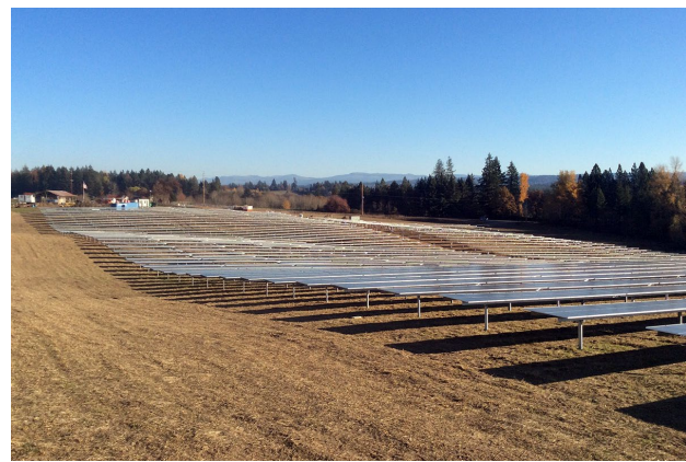
Figure 2: Example Racking System with no tilt.
