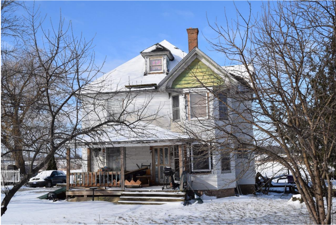
Photograph 17: 2789 Dunsmore Road façade showing multiple alterations resulting in a loss of integrity, looking west.
