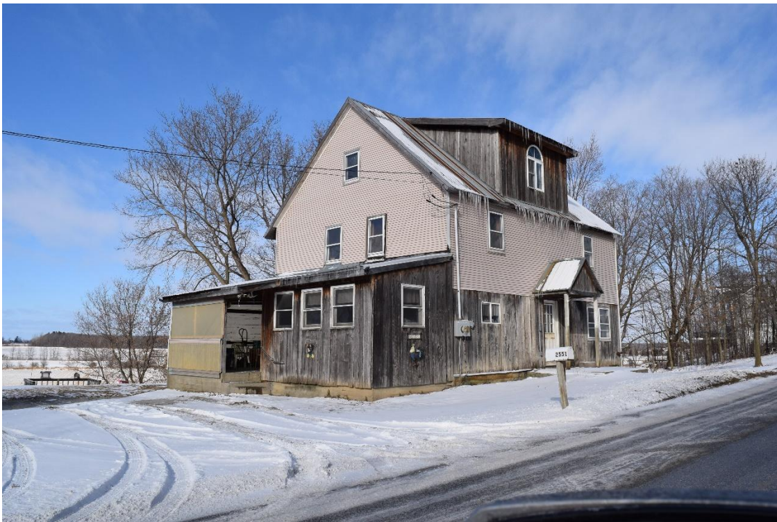
Photograph 8: 2551 Dunsmore Road, looking northwest.
