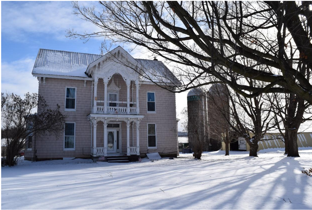
Photograph 11: 2684 Dunsmore Road, looking east-southeast.
