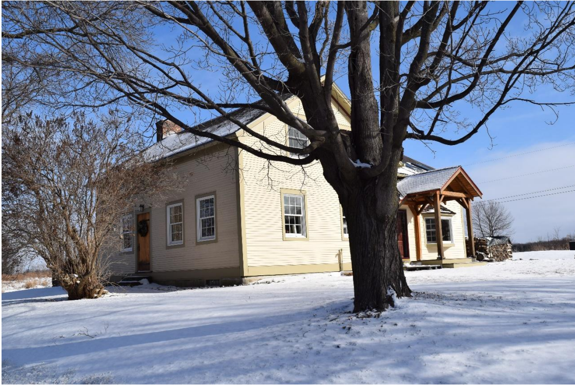
Photograph 5: 2296 Dunsmore Road, looking northeast.
