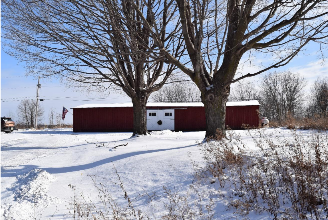
Photograph 7: Barn at 2296 Dunsmore Road, looking east.
