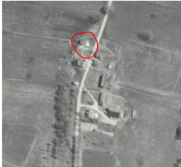
Figure 2: 1962 aerial photograph with 2789 Dunsmore Road circled in red. Note that the two barns across the street have not yet been built. Source: VCGI
