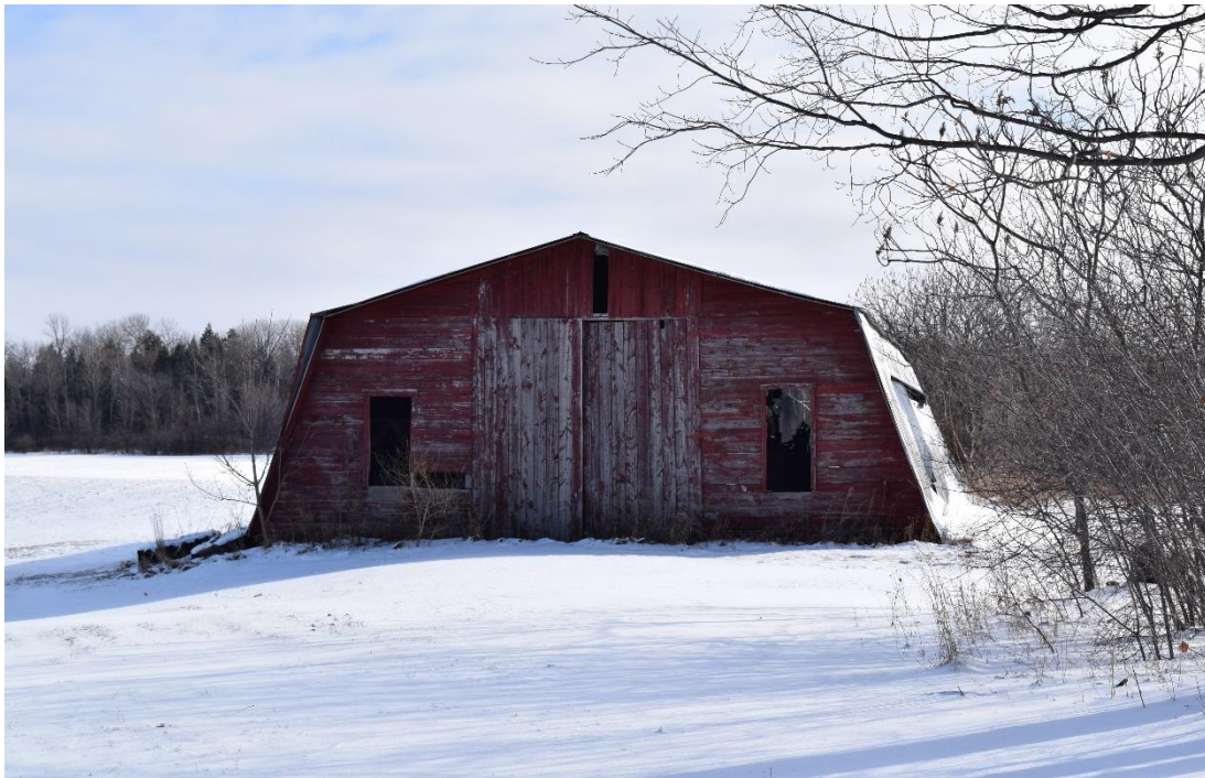
Photograph 12: Barn on the east side of Dunsmore Road historically associated with 2789 Dunsmore Road. It was built sometime after 1966, replacing an older barn that stood here. Currently this barn and the barn in Photograph 13 are located on a separated parcel than the house at 2789 Dunsmore Rd. Looking east.
