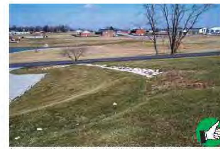
Good construction, seeding, and stabilization of diversion berm. Note that diversion ditch is lined with grass on flatter part of slope, and with rock on steeper part.
