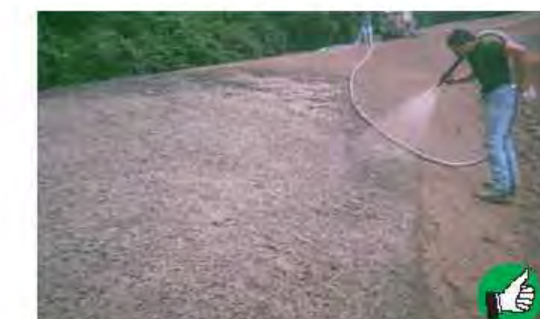
Hydroseeding exposed soil is a good option for stabilizing large areas. Hydroseed is a mixture of seed, fertilizer, water and a tackifier to hold the seed in place before it germinates.
