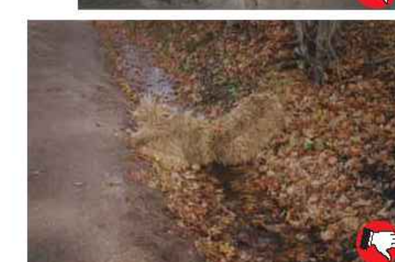
Hay bales must not be used as check dams due to their high failure rates.
