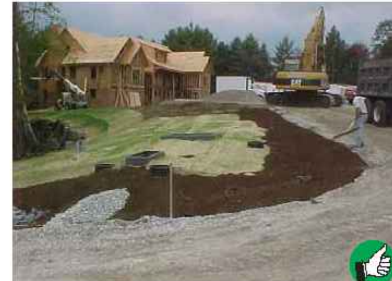
Within 48 hours of final grading, erosion control matting and mulch have been applied.
