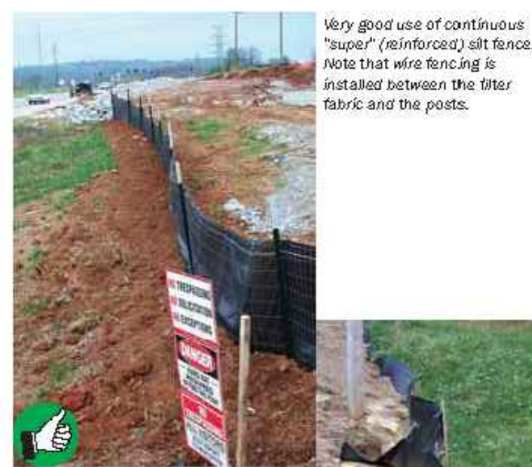
Good use of hook in silt fence to trap sediment in water running along the fence. Sediment must be removed before it reaches halfway to top of fence.
