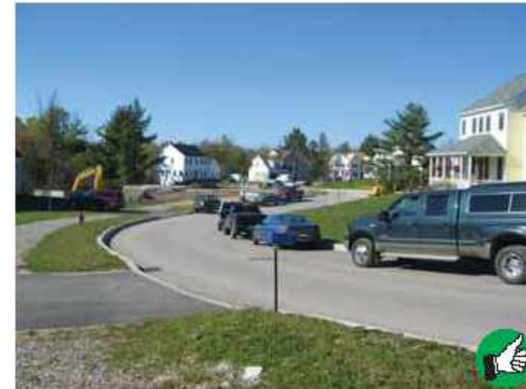
This residential subdivision is being constructed in phases. To limit the total disturbance area, only a few home sites are under construction at one time.
