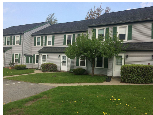
Townhouses and condominiums can offer weatherization opportunities, especially when the development can be addressed as a single project.
