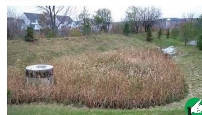
Install all permanent stormwater treatment practices before constructing any impervious surfaces on site. This stormwater wetland treats stormwater runoff from the adjacent parking lot.
