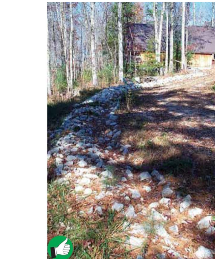
Good installation of rock-lined berm to divert rain runoff around residential construction site on steep slope near a river. Diversion ditches can be lined with grass if channel slopes are 5% or less, and with 4 inch stone if they are steeper.
