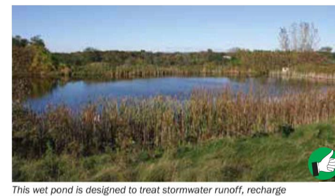
This wet pond is designed to treat stormwater runoff, recharge groundwater, regulate the flow of water into nearby streams, and prevent downstream flooding.
