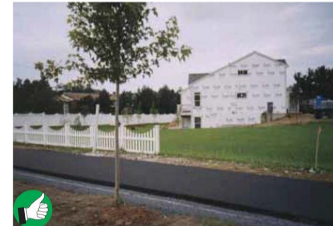
Lawn is fully established before construction is completed at this home site.
