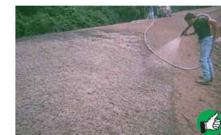
Hydroseeding exposed soil is a good option for stabilizing large areas. Hydroseed is a mixture of seed, fertilizer, water and a tackifier to hold the seed in place before it germinates.
