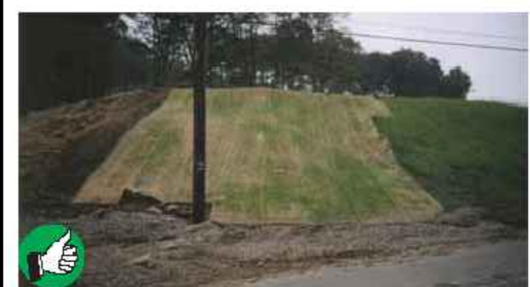
Excellent stabilization of large slopes to limit the area of a disturbance. Make sure to install erosion control matting within 48 hours of grading to ensure good contact between soil and mat.
