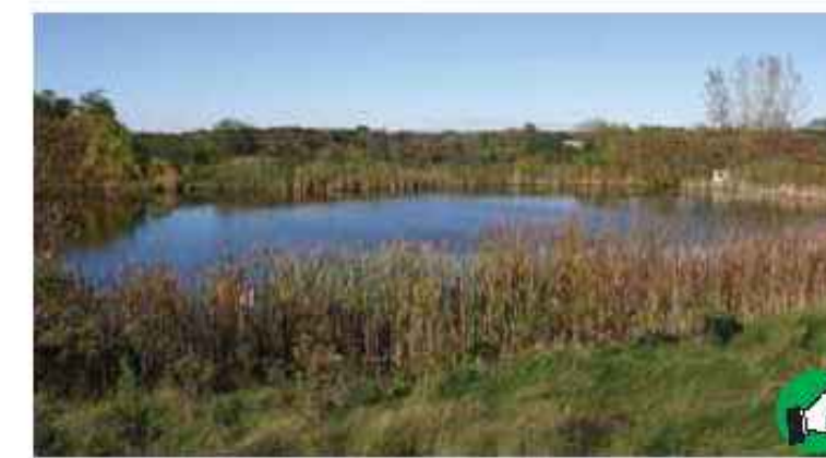
This wet pond is designed to treat stormwater runoff, recharge groundwater, regulate the flow of water into nearby streams, and prevent downstream flooding.
