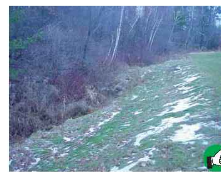
Stabilization and seeding of slopes before winter will reduce or eliminate erosion in the spring. The grass on this slope is holding the soil in place and promoting infiltration of the melting snow.
