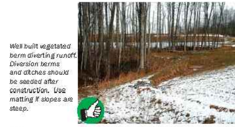
Good construction, seeding, and stabilization of diversion berm. Note that diversion ditch is lined with grass on flatter part of slope, and with rock on steeper part.
