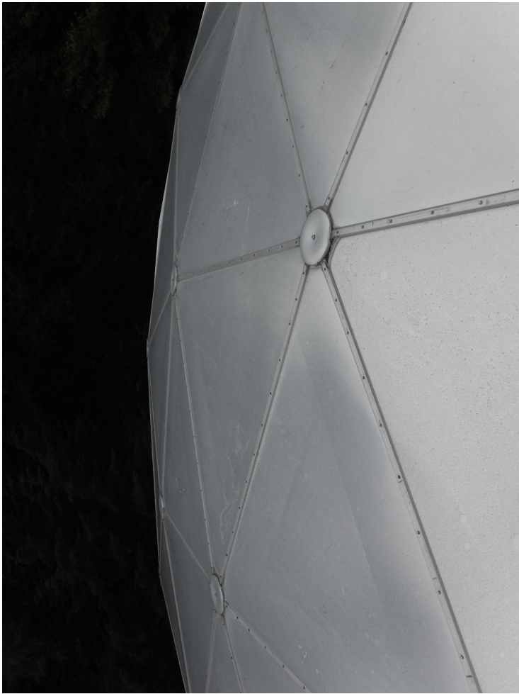
Exterior roof panels (1)
