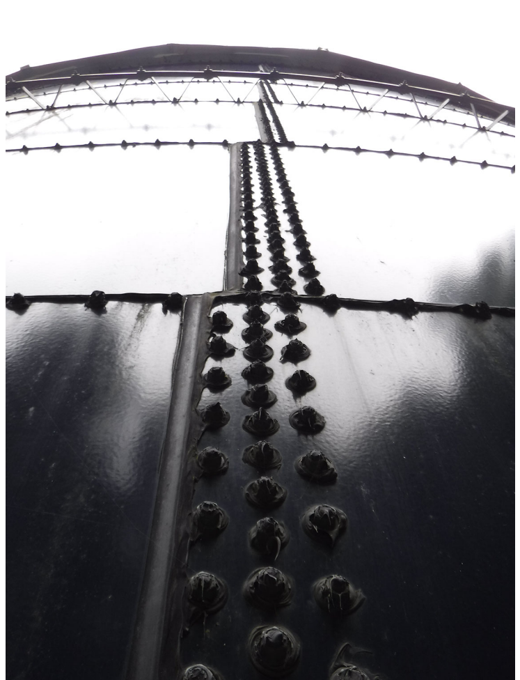
Exterior vertical seam
