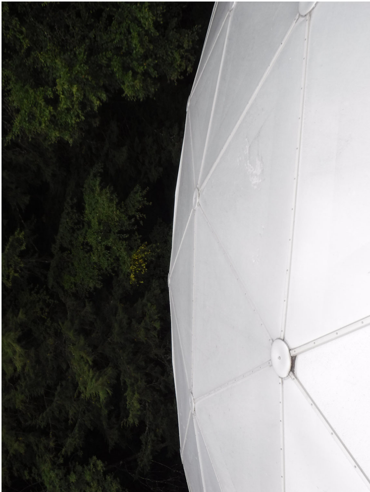
Exterior roof panels (3)
