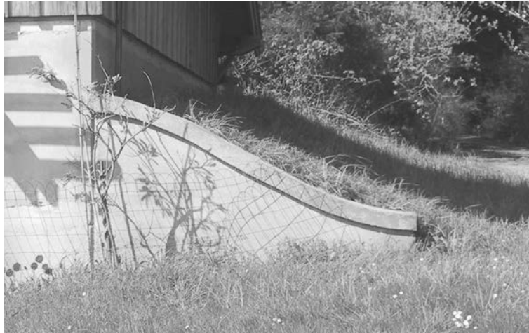
21.19 Rammed Earth buttress/ retaining wall.
