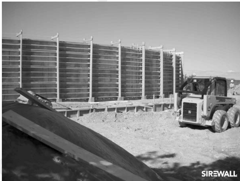
24 25 26 27 28 29 30 31 32 33 34 35 36 37 38 39 40 41 42 43 21.18 Common SIREWALL forming system.
