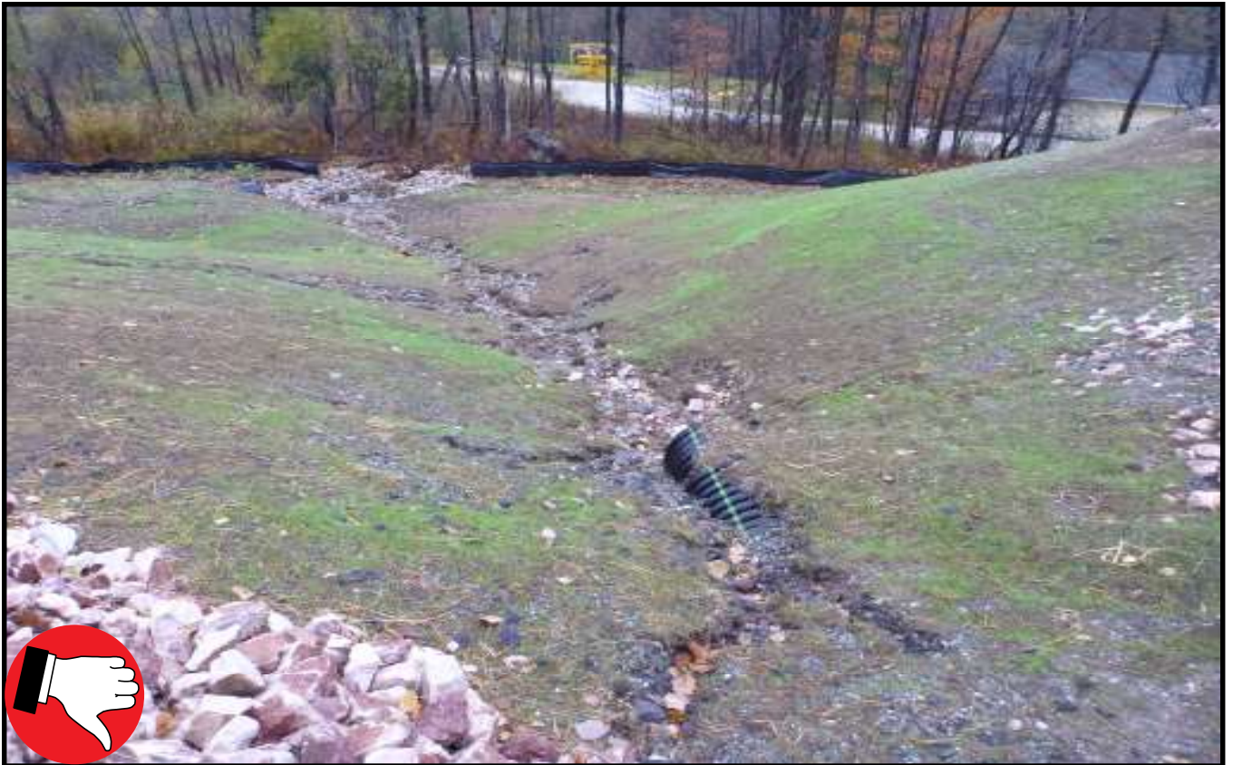
Before installing rock outlet protection
