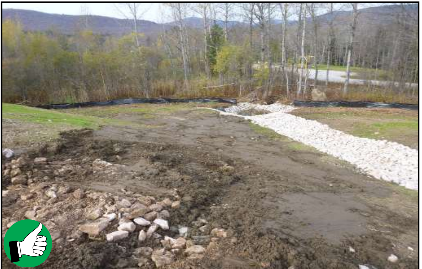
After installing rock outlet protection
