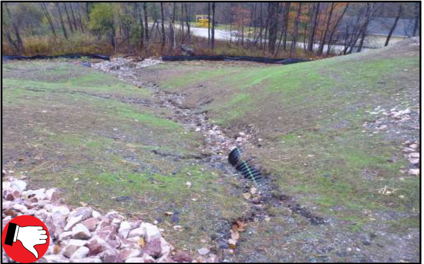
Before installing rock outlet protection
