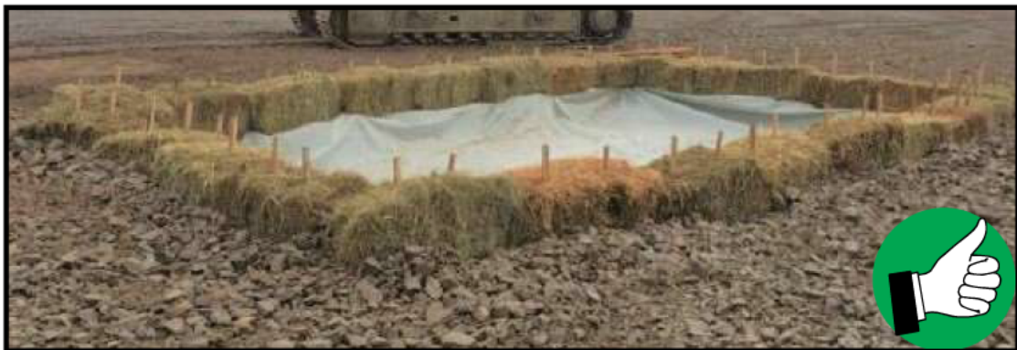
ABOVE GRADE STRAW BALE CONCRETE WASHOUT DETAIL
