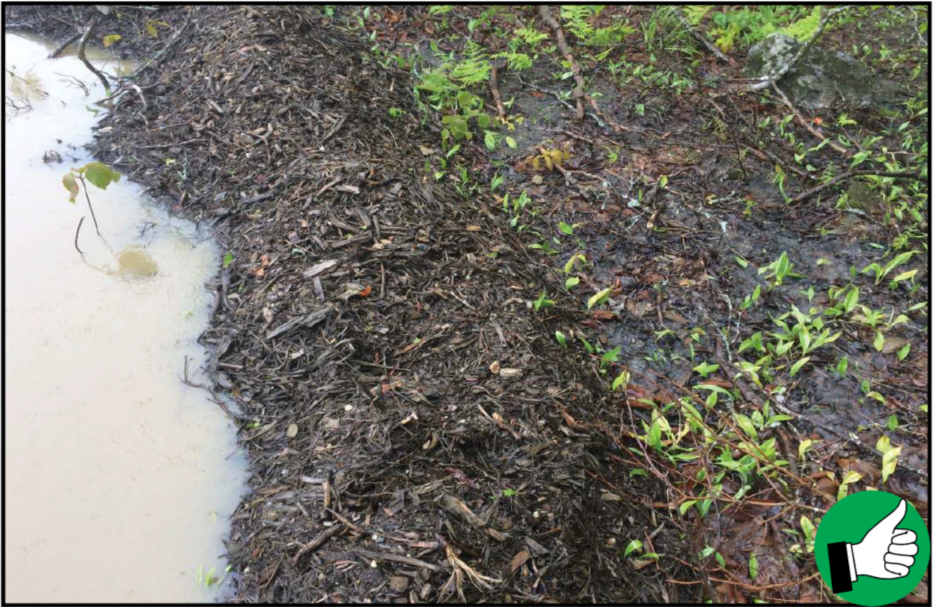
The erosion control berm above is allowing for both ponding and filtering of stormwater.
