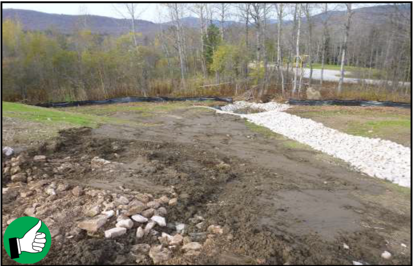
After installing rock outlet protection
