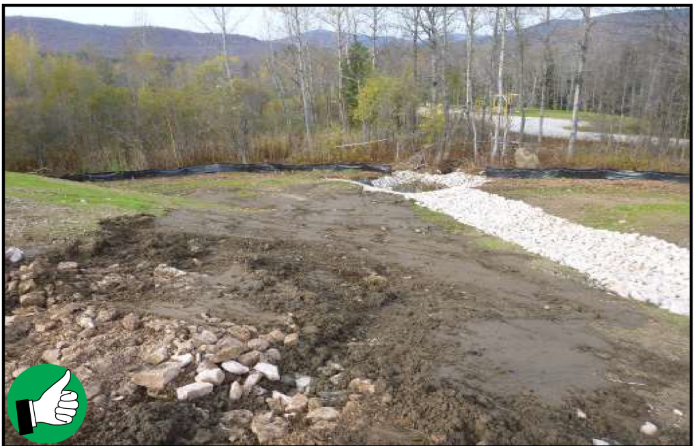
After installing rock outlet protection
