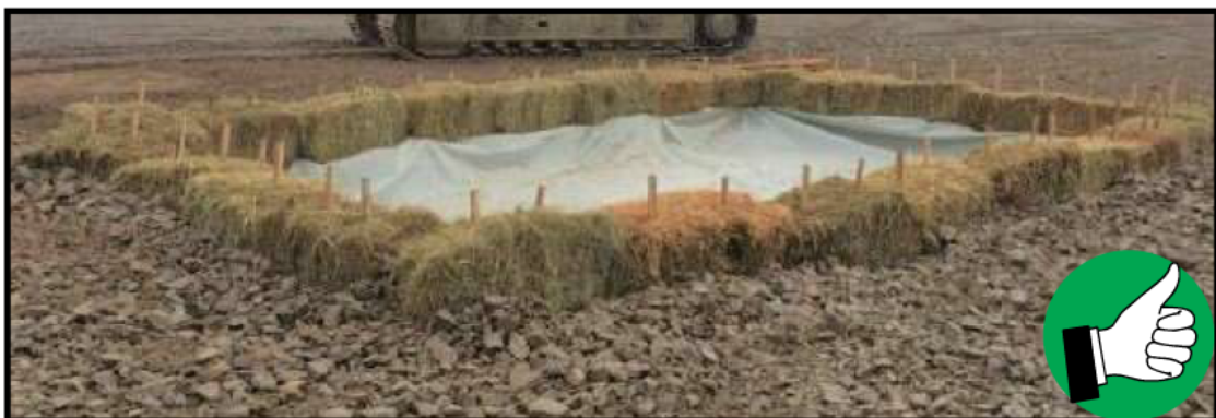
ABOVE GRADE STRAW BALE CONCRETE WASHOUT DETAIL
