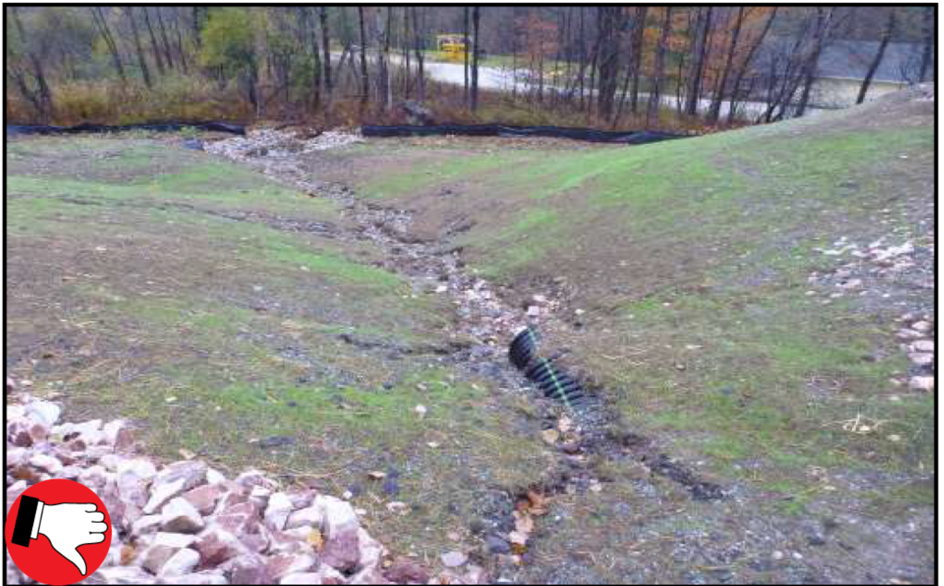
Before installing rock outlet protection
