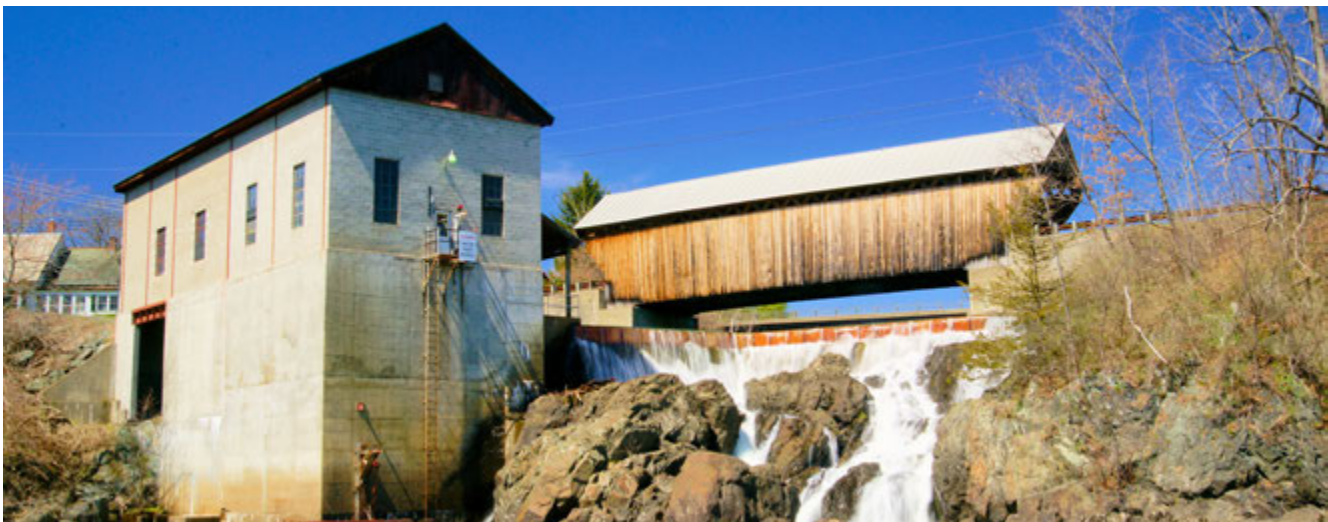
Willard Bridge, Hartland | © John Knox
