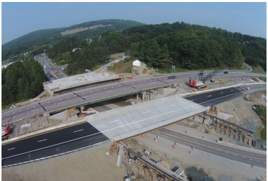
Hartford I-91 Bridge | © EIV Technical Services
