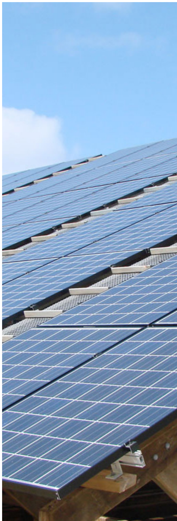
Solar panels | Source: Unknown
