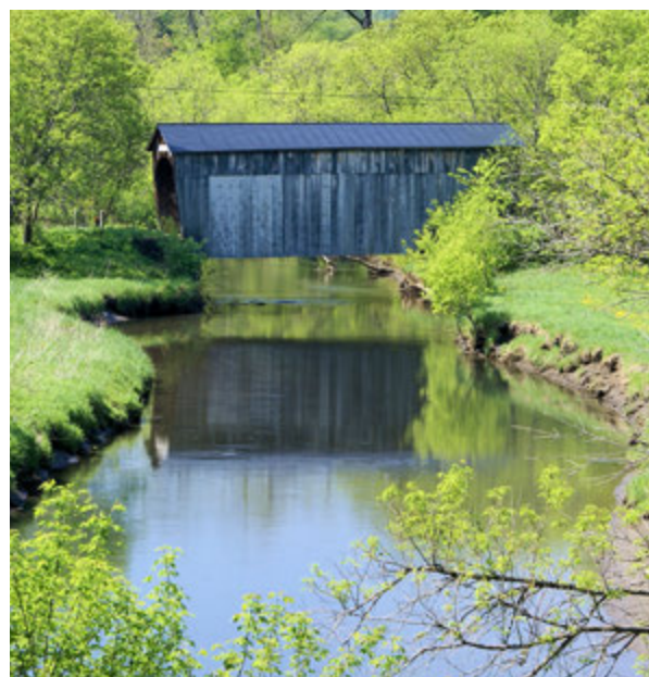
Kingsbury Bridge, Randolph | © John Knox
