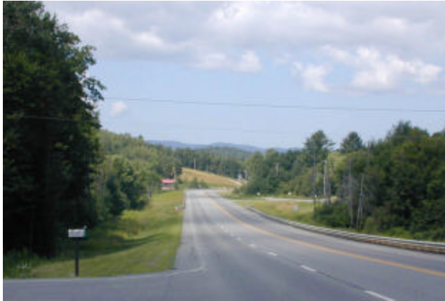
Photo 2: Route 9 Looking West by Molly Stark State Park (7.4 miles) Existing turbines are on distant ridge looking ahead and right; proposed eastern ridge turbines would be ahead and left.
