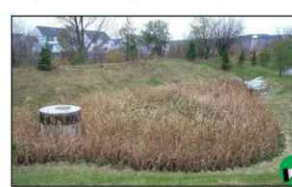
Install all permanent stormwater treatment practices before constructing any impervious surfaces on site. This stormwater wetland treats stormwater runoff from the adjacent parking lot.
