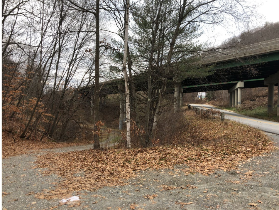
Photo 2— At the site entrance from River Road South, view is west. Interstate overpass is north of the Project array. The Project site is 1340+ feet generally west of this location, completely out of view.
