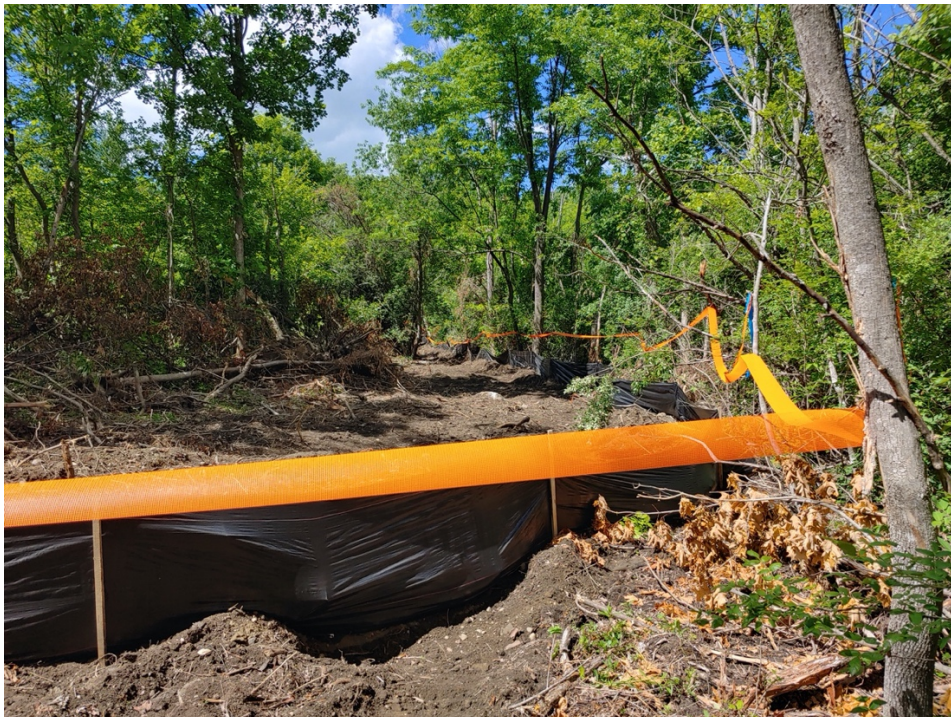
Photo #8 Standing in northeast corner RTE #2 looking north
