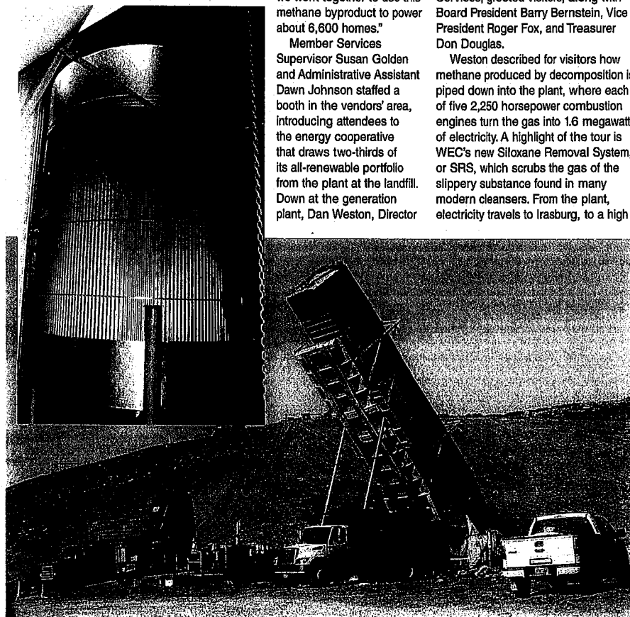
(inset) WEC's new Siloxane Removal System dramatically improves the performance of its five 1.6 megawatt engines.
