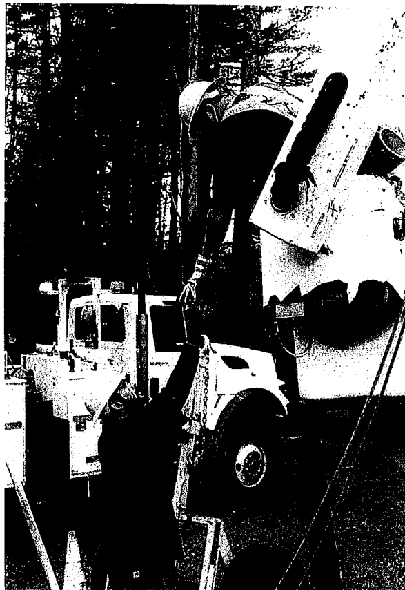
Donnie Singleton (L) and Larry Gilbert (in bucket) setting a broken pole in Middlesex.
