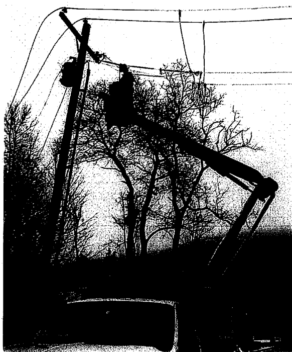
At right: Note the dangling wires on the left side of the pole. Below: Saturated ground, big pines, and high winds are a bad combination for poles and wires.
