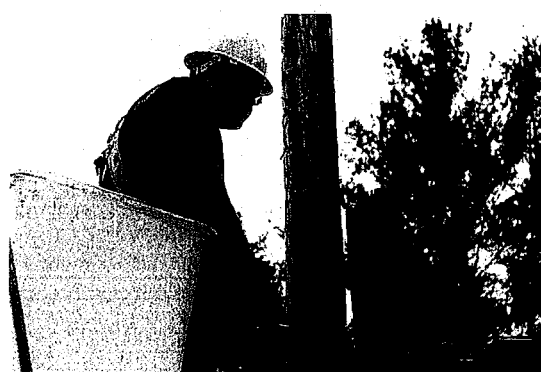
Larry Gilbert, First Class Lineworker, works to set a new pole next to one broken by the windstorm. WEC replaced 19 broken poles in all.
