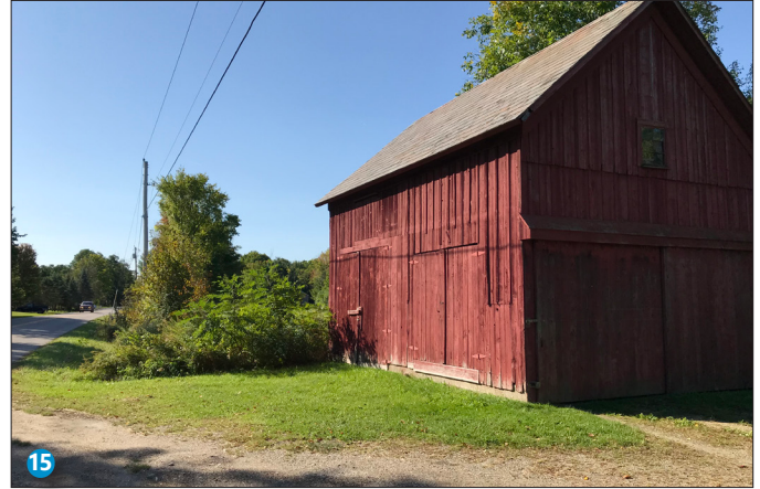
Photo 15: View from Shard Villa Road looking south at an existing outbuilding along the road.
