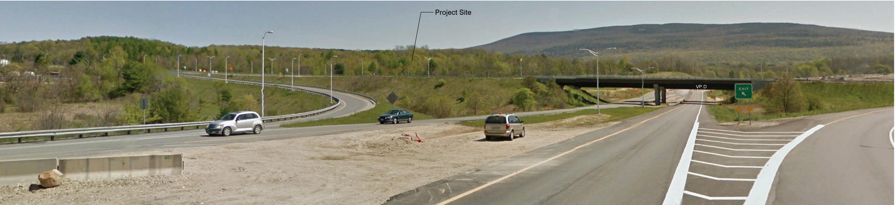
C - VIEW LOOKING NORTHEAST FROM THE EASTBOUND ROUTE 279 / ROUTE 7 INTERCHANGE TOWARDS THE PROJECT SITE
