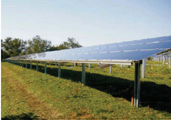
A fixed panel solar array such as this one is planned for construction in Pownal in 2012. It will include 370 solar arrays covering 12 acres of land and produce 2.2 MW at capacity.
