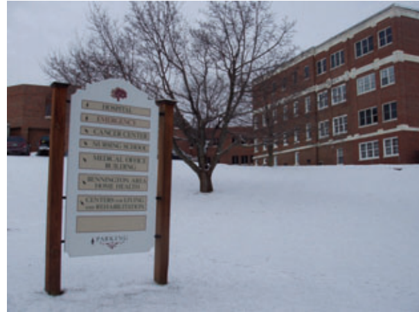
The main campus of the Southwestern Vermont Health Care uses a lot of energy; planned improvements could significantly reduce energy costs.
